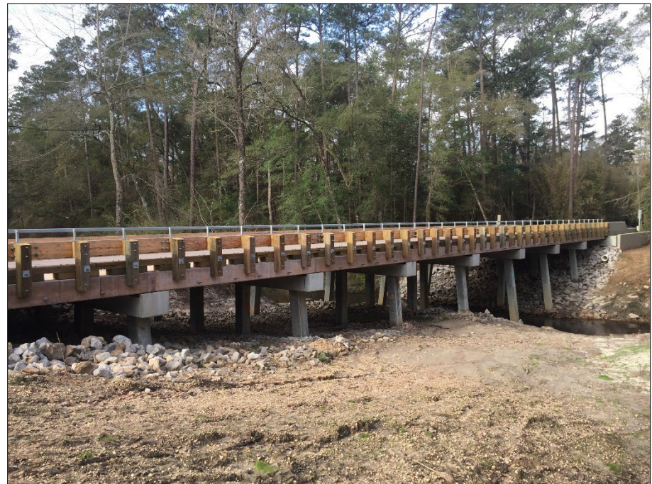
Aesthetic Concrete Slab Span Bridge designed by Forte and Tablada
