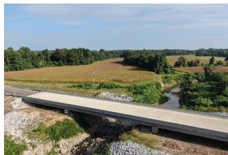
New 3-Span Bridge with FIB Girders
