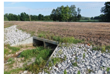
New 2-Span Culvert
