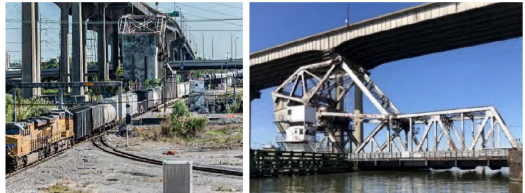
Almonaster Avenue Bridge
