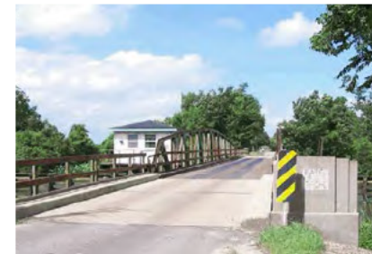
Bayou Teche Swing Bridge
