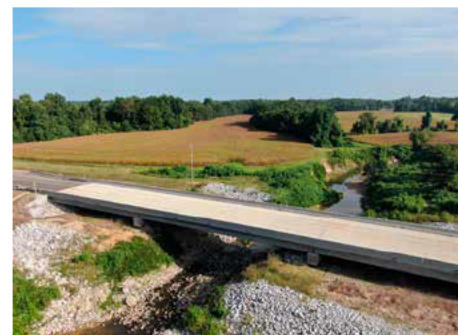
New 3-Span Bridge with FIB Girders
