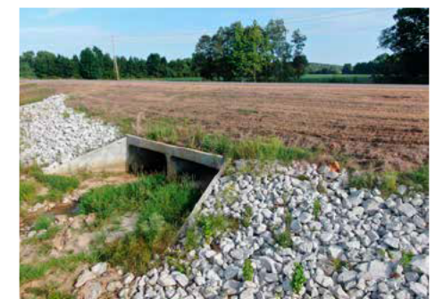
New 2-Span Culvert
