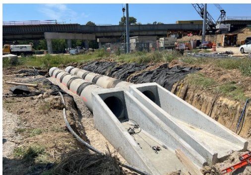
Installation of Culverts and Safety End Treatment - College Dr
