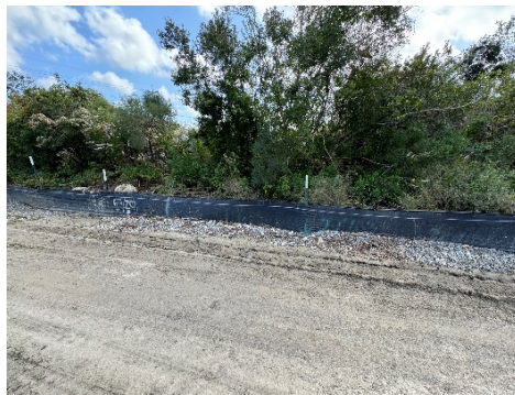
Inspection of Project Silt Fencing LA302
