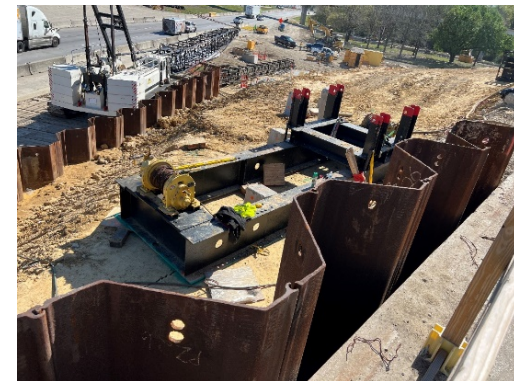
Sheet Pile Retaining Wall - College Dr.
