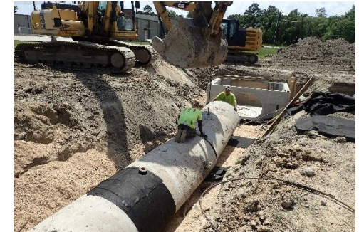
Major corridor subsurface drainage improvements at existing intersections, including design, construction administration, and construction oversight of large-diameter storm drainage systems.
