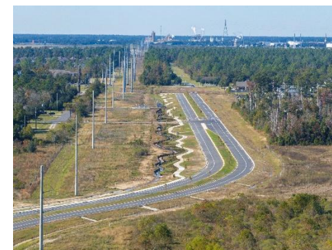
Completed roadway featuring landscaped medians that enhance both roadway safety and corridor aesthetics.
