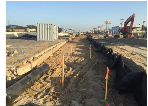
Split-phase construction of the two-way frontage road system accommodated dense commercial development and significant utility conflicts—experience directly relevant to minimizing construction impacts along LA 384.
