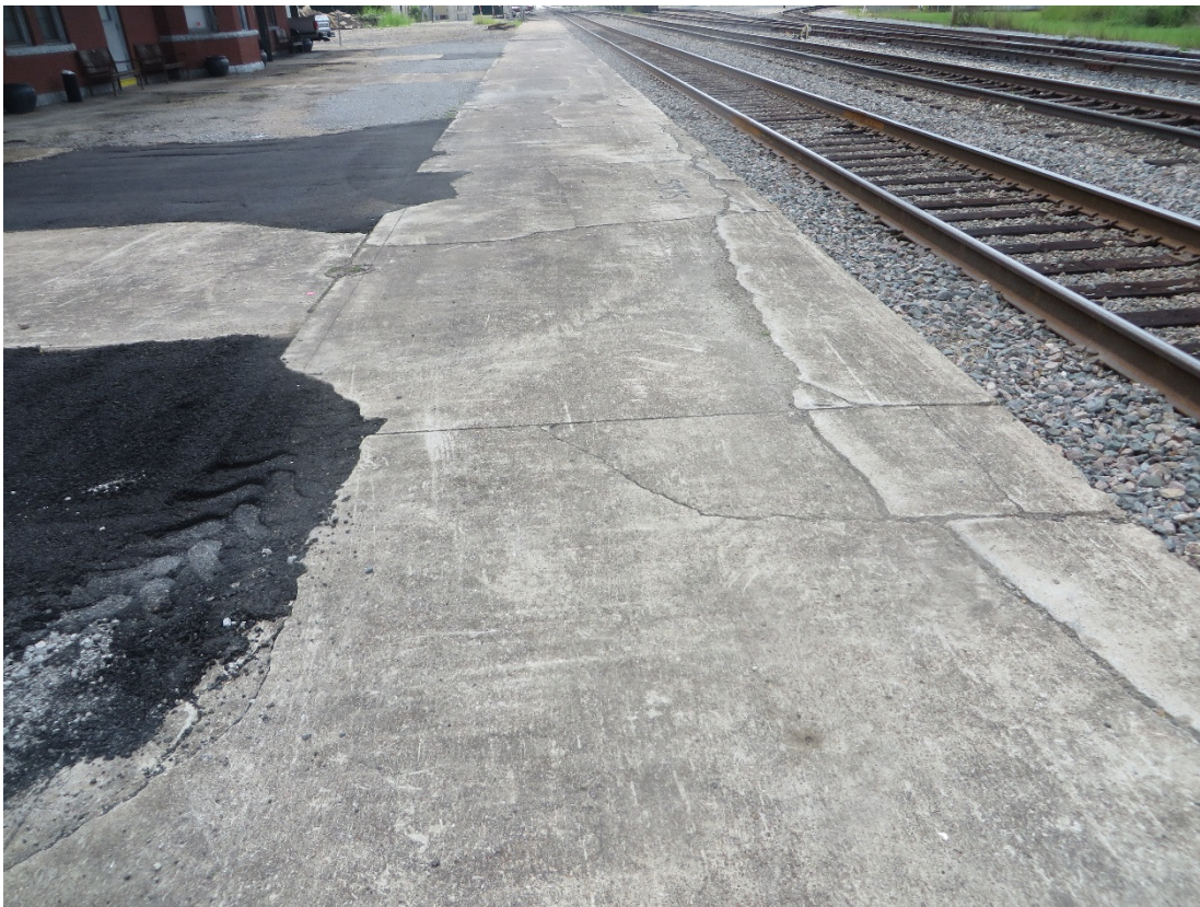
Figure D-4. Asphalt repairs adjacent to deteriorated platform (looking southeast).
