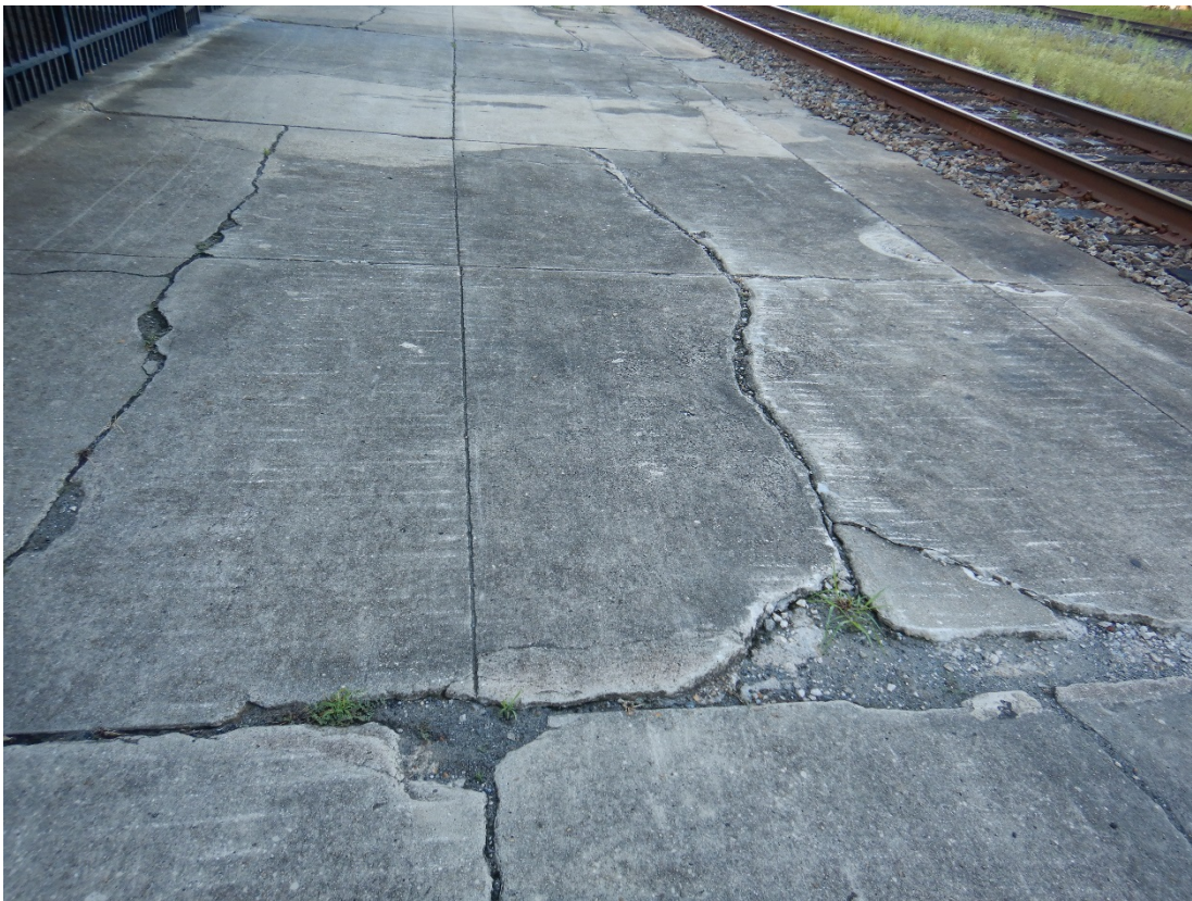
Figure G-2. Cracked concrete platform without tactile warning surface strip.
