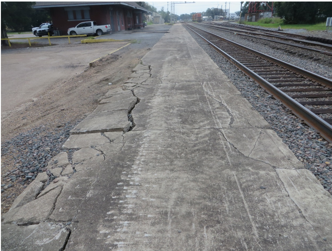
Figure D-2. Concrete failure on platform (looking southeast).
