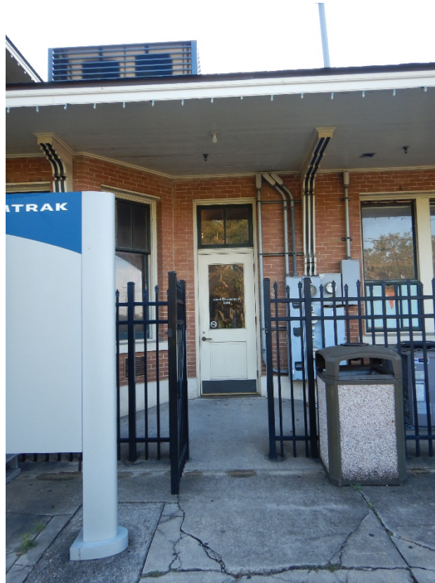
Figure G-7. Entrance from platform to Amtrak waiting room (looking east). Gate opening is 36 inches wide and door opening is 34-1/2 inches wide.
