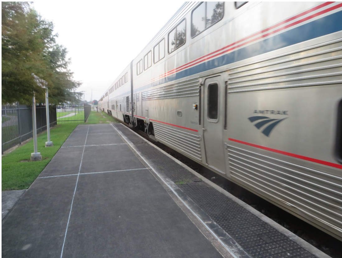
Figure C-1. Platform (10 feet x 370 feet) with tactile warning surface (looking northwest).
