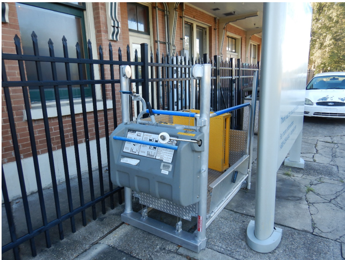
Figure G-6. Wheelchair lift on platform; no enclosure provided (looking southeast).
