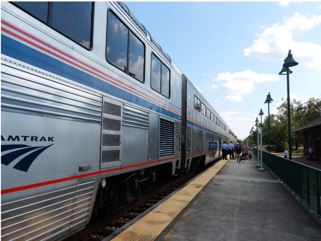
Figure F-2. Overall condition of platform (15 feet x 557 feet) including lighting (looking south).
