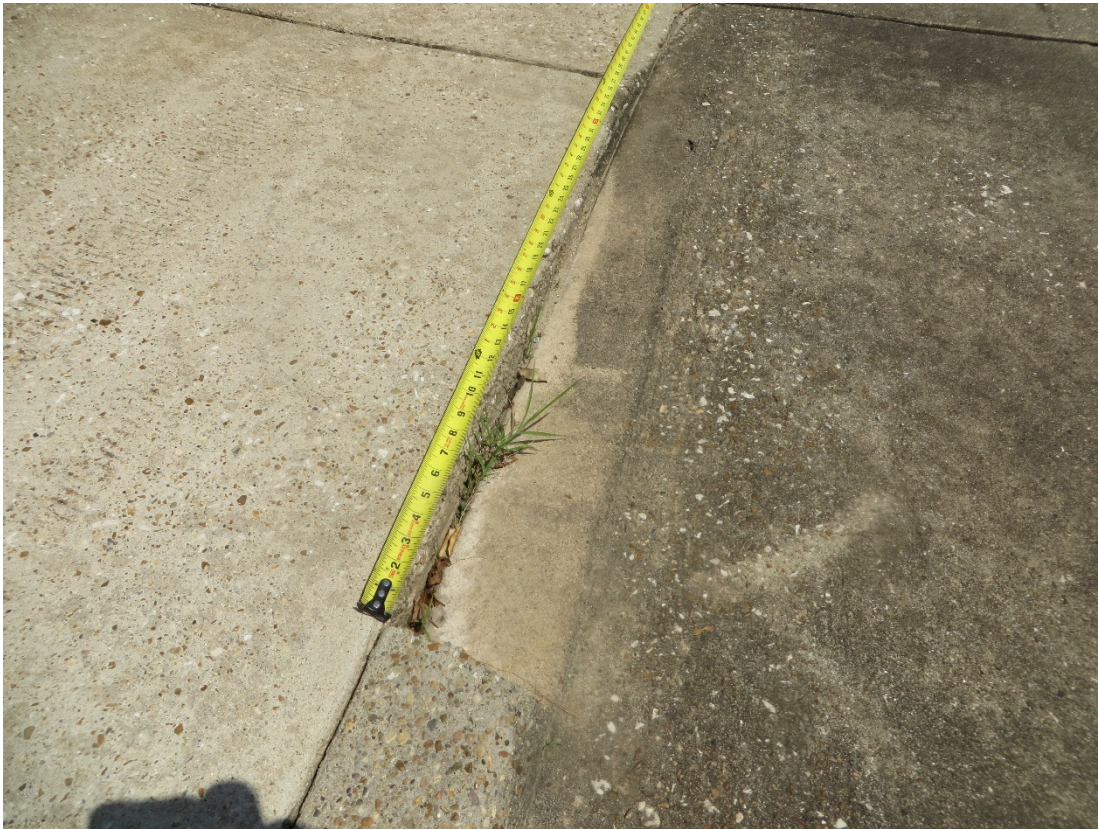
Figure B-25. Deteriorating concrete at joint on west side of building (approx. 3 feet long) leading to building entrance.
