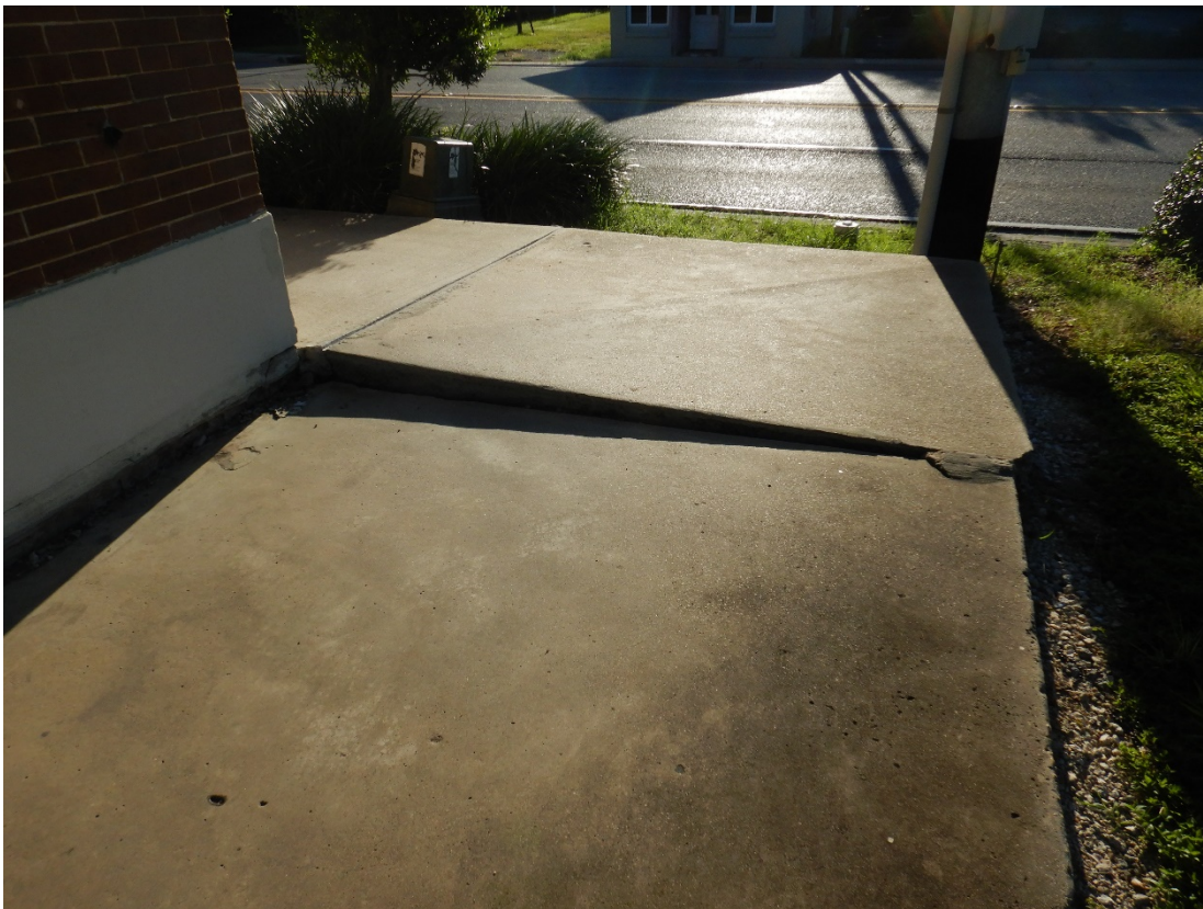
Figure G-16. Concrete walkway around southeast corner of building has settled 4 to 6 inches making the route inaccessible for wheelchairs (Front Street in background).
