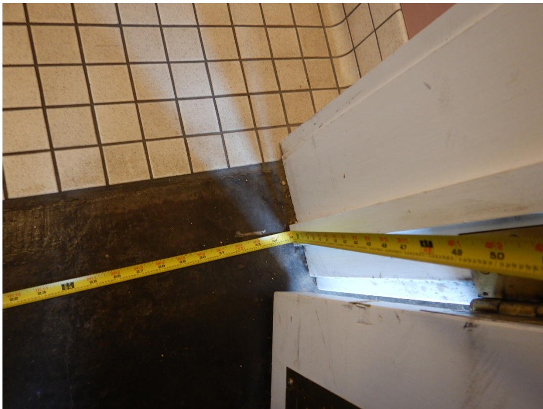
Figure F-16. Restroom door frame measures 35 inches wide; door opening width is less.
