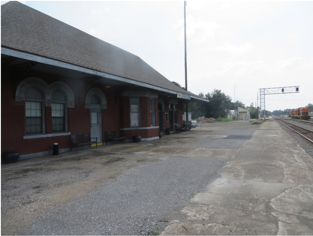
Figure D-3. Deteriorated platform condition adjacent to building (looking southeast).
