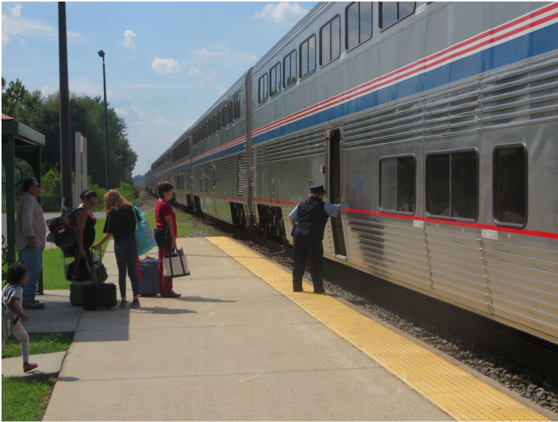
Figure B-1. Platform (15 feet x 170 feet) with ADA compliant tactile strip. West end of platform.
