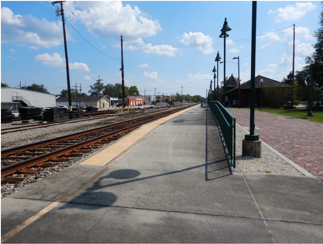
Figure F-1. North edge of platform with ramp for wheelchairs and historic-style lighting on platform (looking south).
