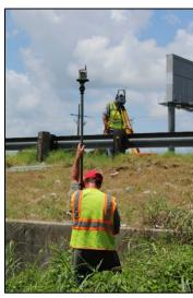
project along LA 415. This work included using 3D Scanning for the bridge at I-10 bridge @ LA 415 as well as scanning every 500' for control verification and incorporation of the Mobile Lidar for the I-10 pavement.
