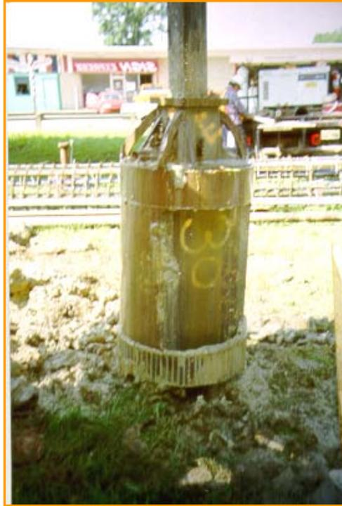
**Figure A-1: Drilled Shaft Cleanout Bucket**
