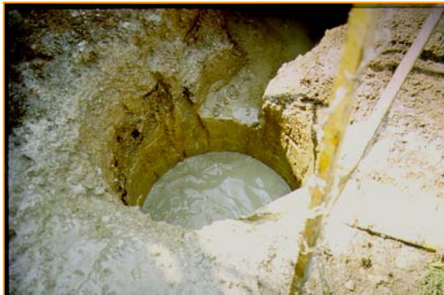
**Figure A-7: 3' Drilled Shaft Hole with Bentonite Slurry in hole.**
