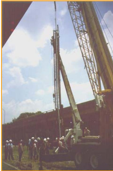
**Figure A-20: The reinforcing cage is lifted into place with the crane.**
