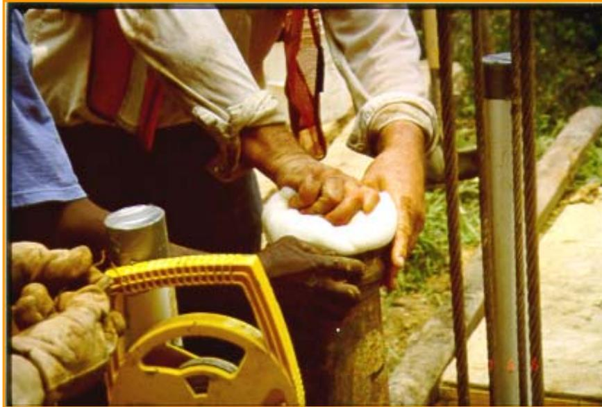
**Figure A-16: Installing the PIG in the Tremie Pipe**
