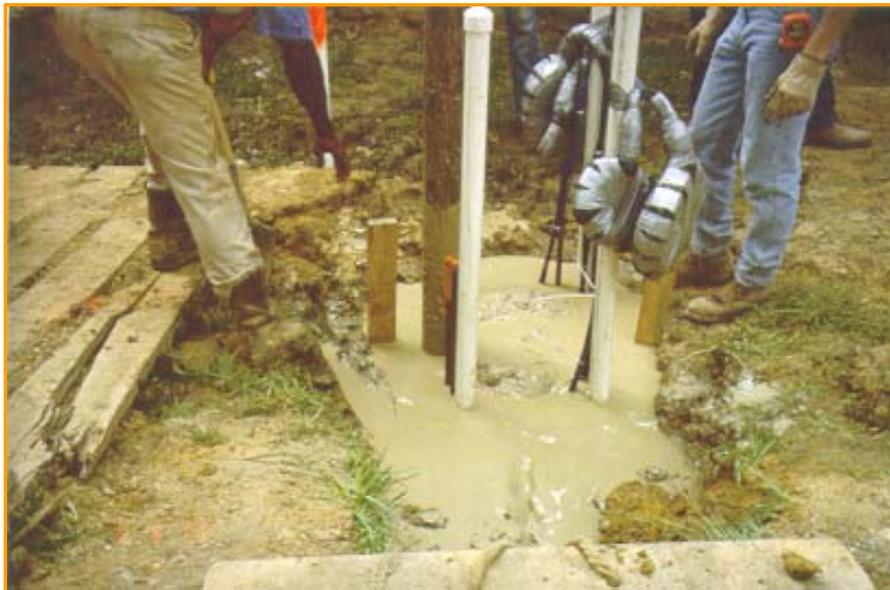
**Figure A-17: View on top of test shaft as the rising concrete approaches the surface.**
