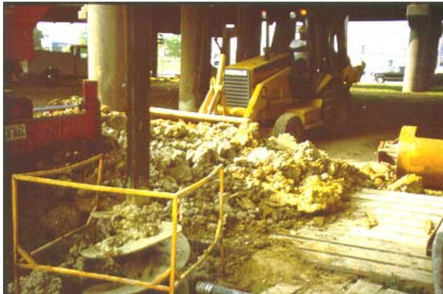
**Figure A-9: The front-end loader removes excavated material while the Kelly Bar places the auger in the hole.**
