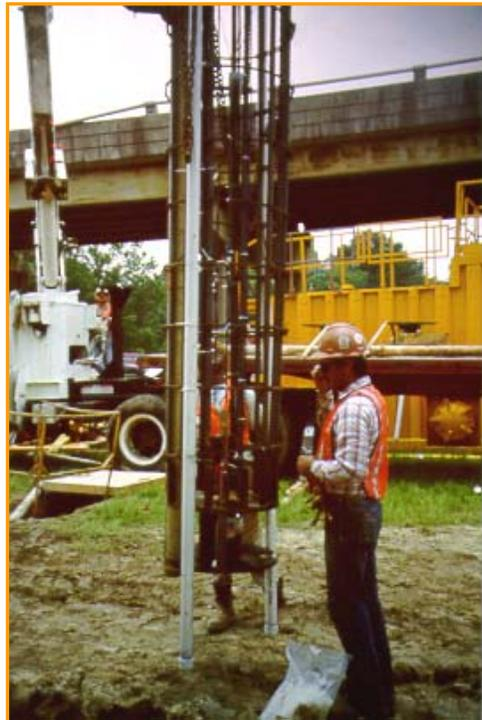
**Figure A-4: 3' Diameter Test Drilled Shaft**
