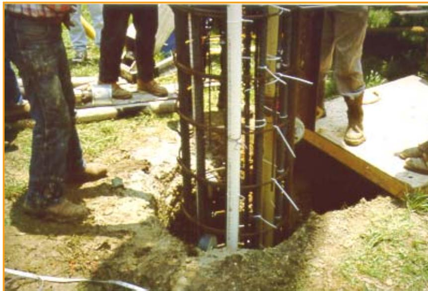
**Figure A-21: The Drilled Shaft reinforcing cage and access tubes are lowered into the shaft.**
