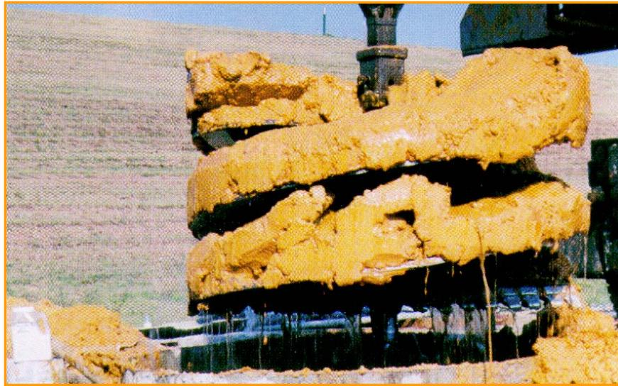
**Figure A-8: Drilling shaft with polymer slurry.**
