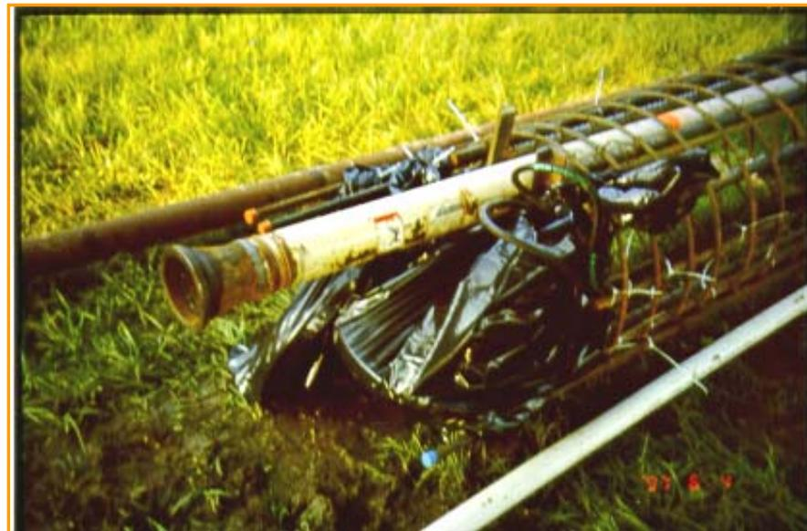
**Figure A-11: Tremie Pipe and Test Shaft instrumentation.**
