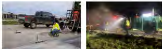
US 90 construction operations: slab jacking (left) and asphalt overlay (right).
