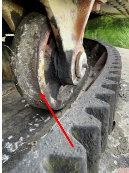
Figure 3-42: Balance wheel and track, note corrosion, and surface quality of the balance wheel.
