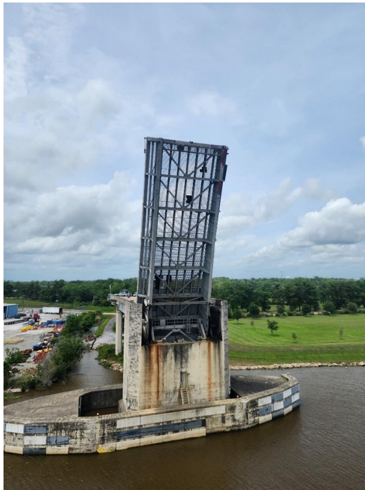
Figure 5-1: Bascule pier with a pier protection system.
