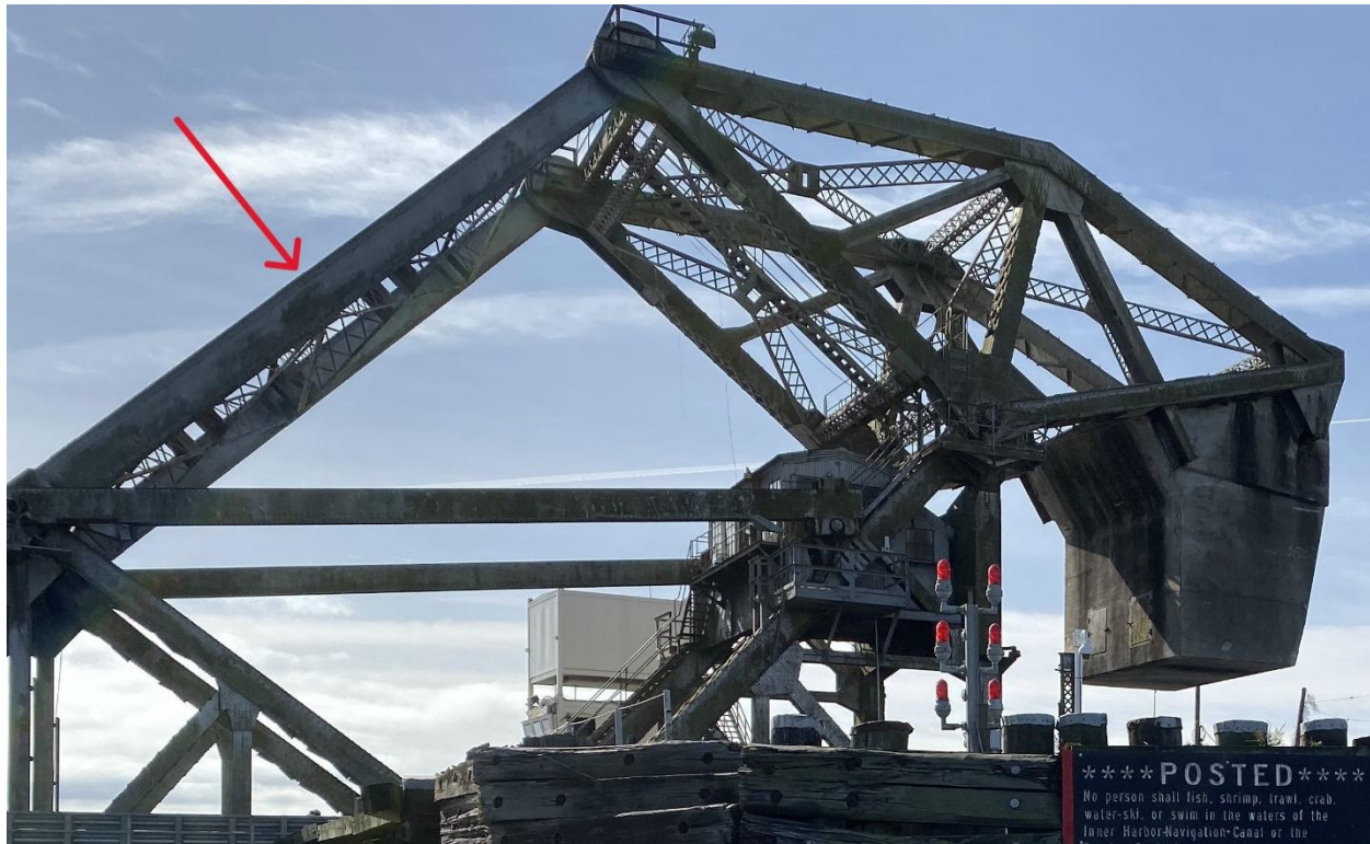
Figure 5-8: Link on Strauss bascule bridge.
