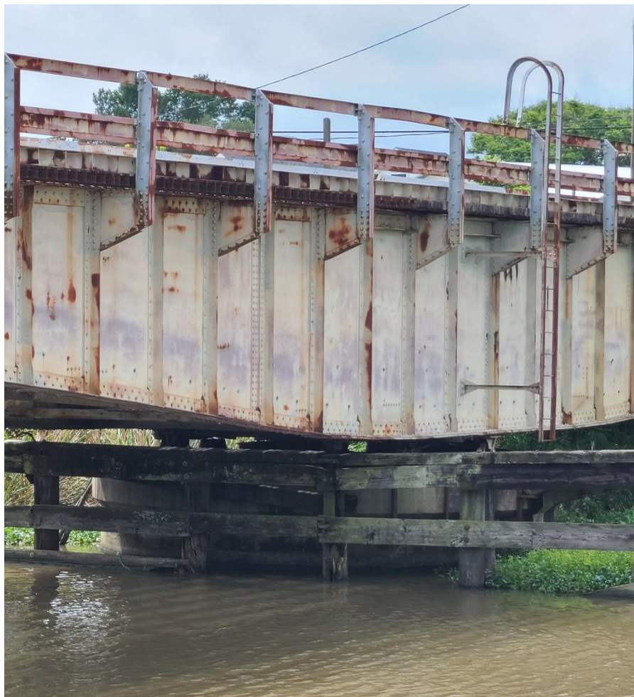
Figure 5-2: Swing bridge pivot pier with pier protection system
