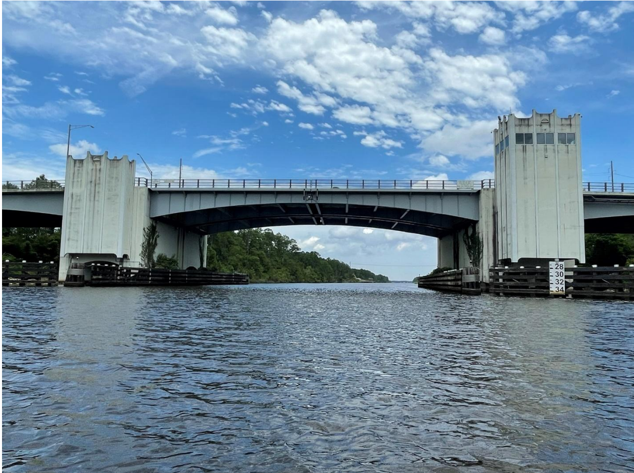
Figure 2-26: Double-leaf bascule bridge.
