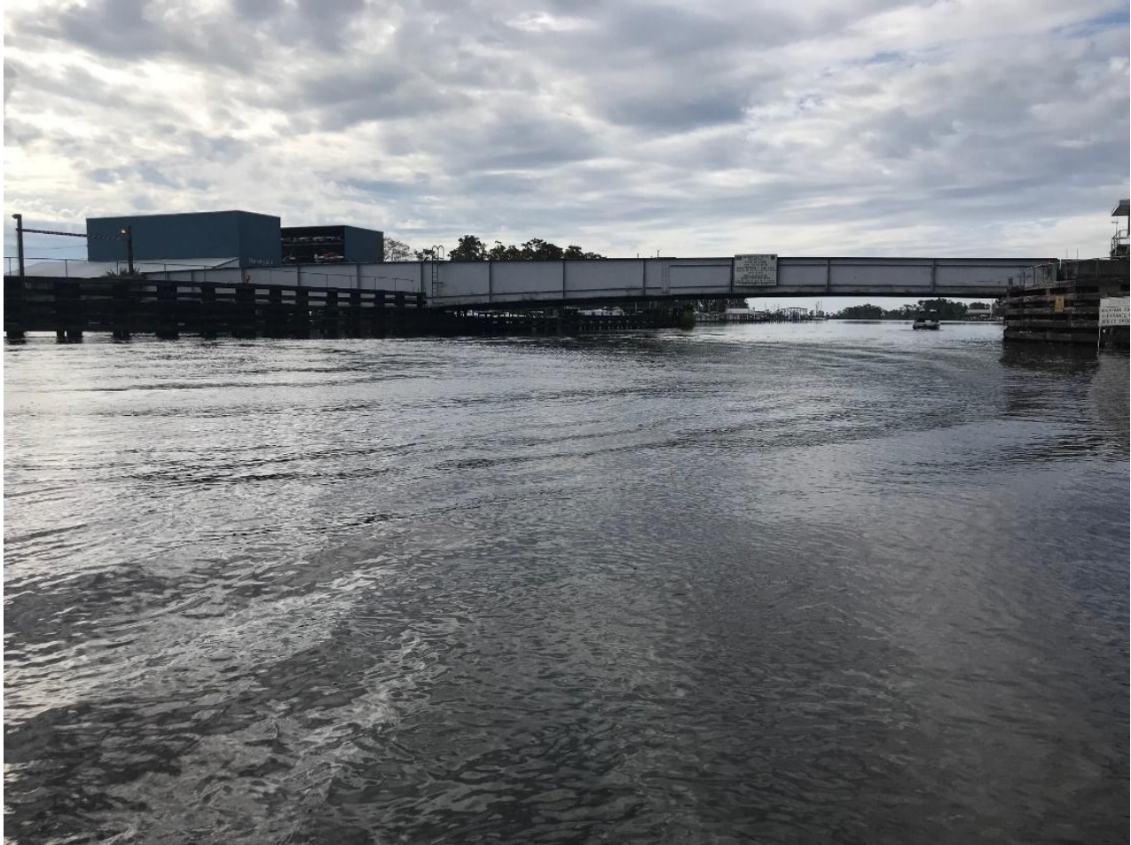
Figure 2-5: Bob-tailed swing span bridge.
