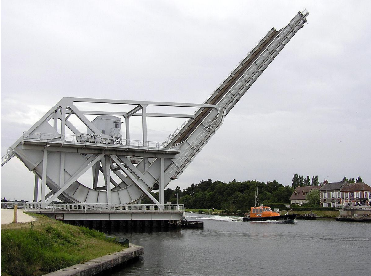
Figure 2-31: Rolling lift bascule bridge.
