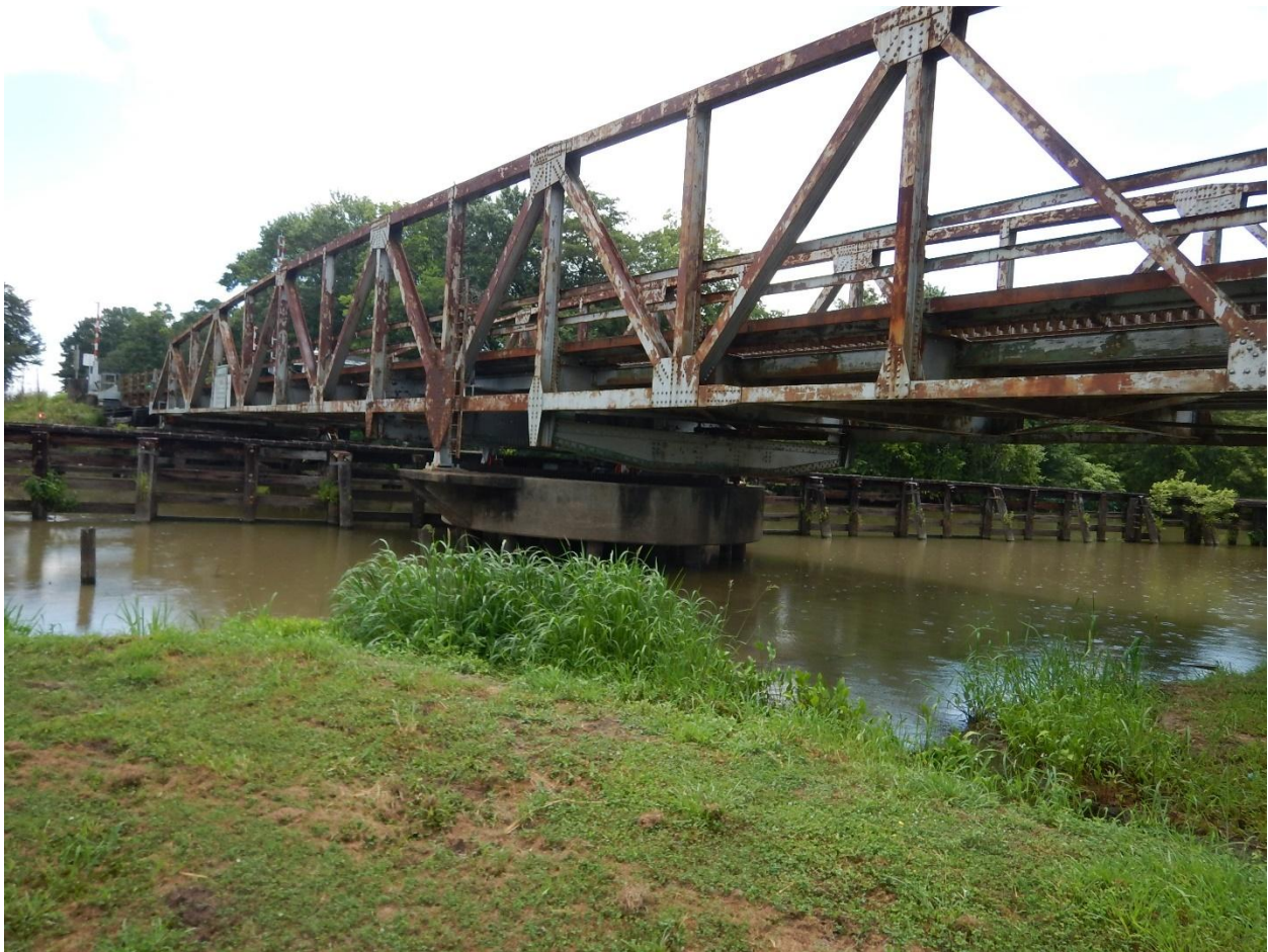
Figure 2-3: Symmetrical truss span swing bridge.
