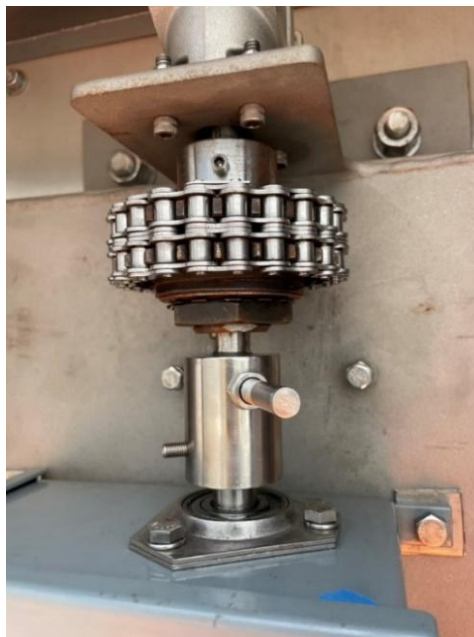
Figure 3-9: Chain coupling of a rotary limit switch with no observable defects.
