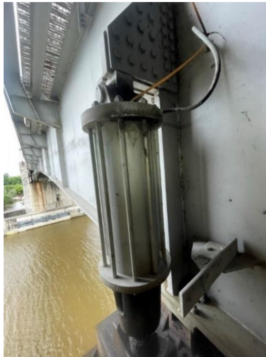
Figure 3-32: Bascule bridge buffer cylinder.
