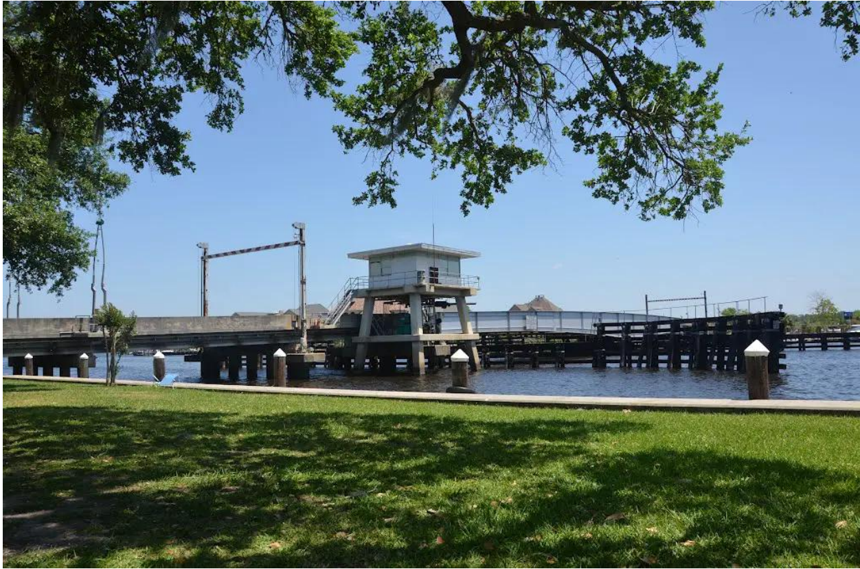
Figure 2-2: Swing bridge in Madisonville over the Tchefuncte River.
