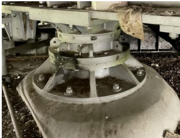
Figure 3-39: Center bearing of a swing bridge.
