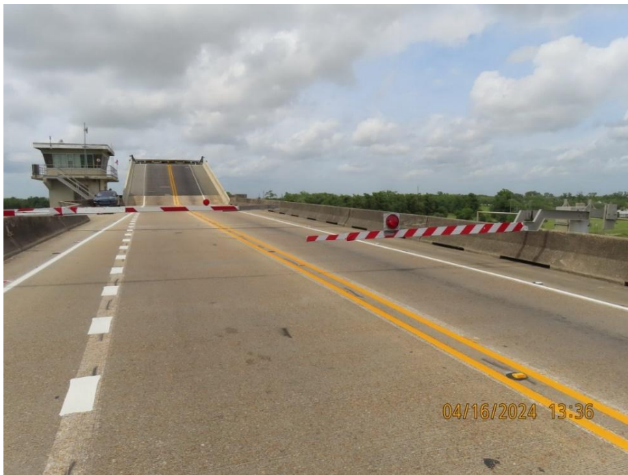
Figure 4-28: Traffic gates in the lowered position.
