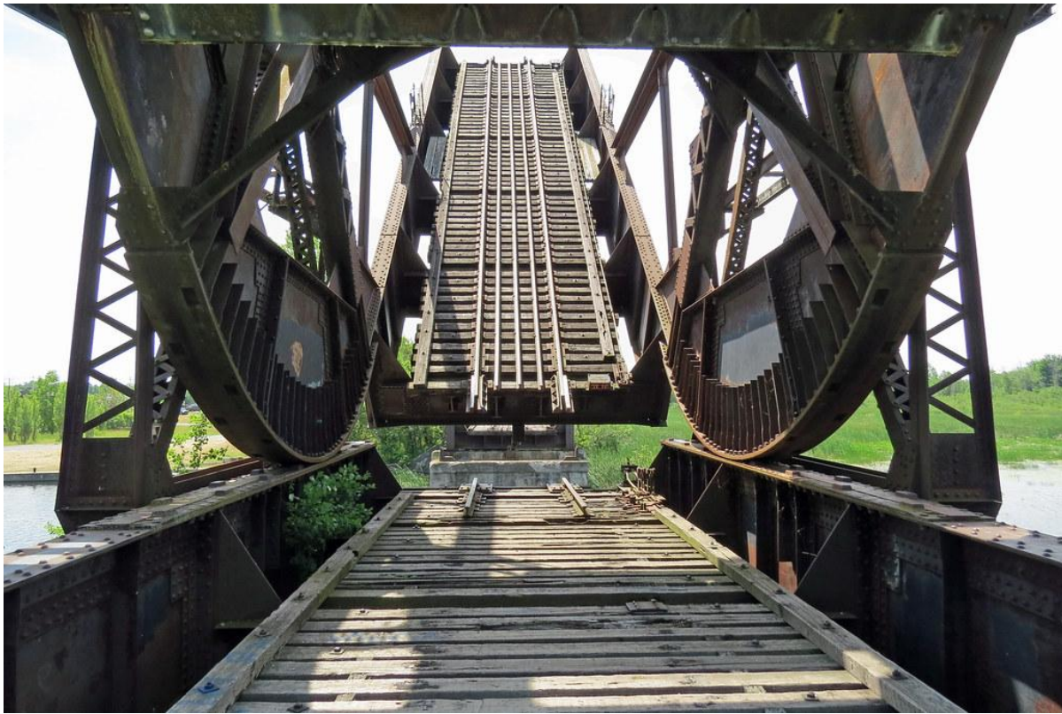
Figure 5-5: Rolling lift track girders on bascule bridge.
