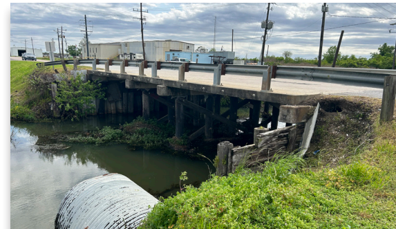
Photo showing existing erosion pipes, retaining walls, overhead electric facilities and bankline erosion at bridge site. (3/26/2024)
