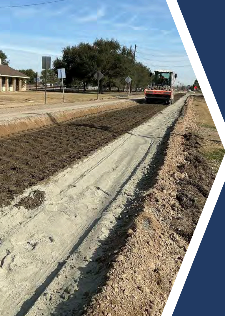
LA 95 & LA 1100 Improvements - Roadway Base Preparation
