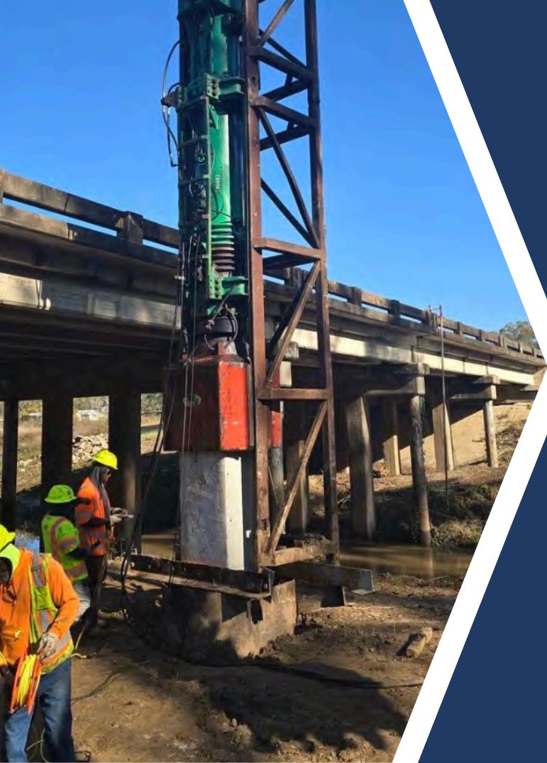
Bayou Carron Bridge Project - Bridge Foundation Construction
