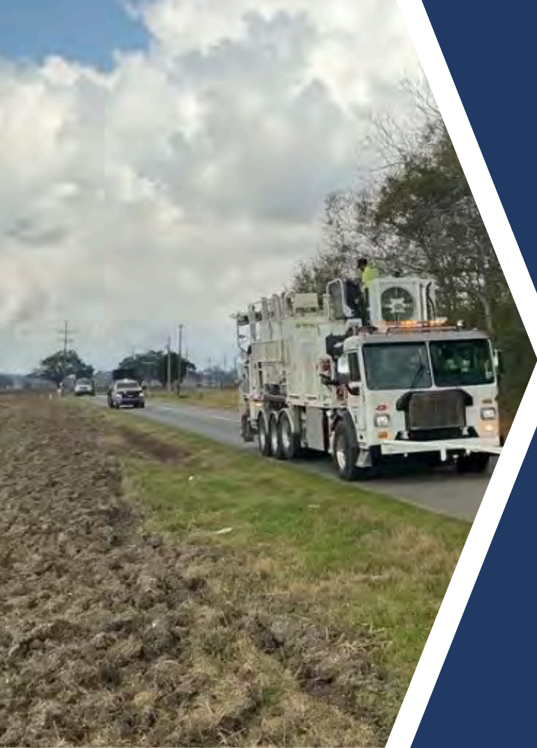
St. Mary Parish Signing & Striping Project - Pavement Marking Operations
