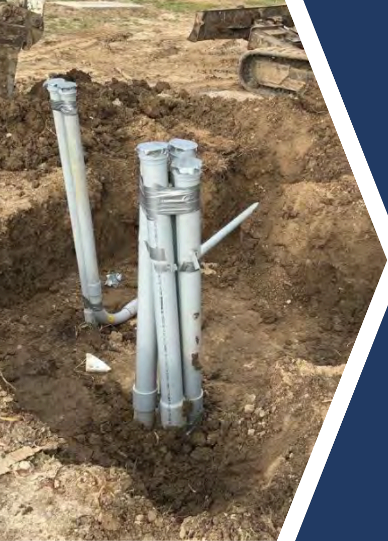
Lafayette FYA Project - Traffic Signal Conduit Installation
