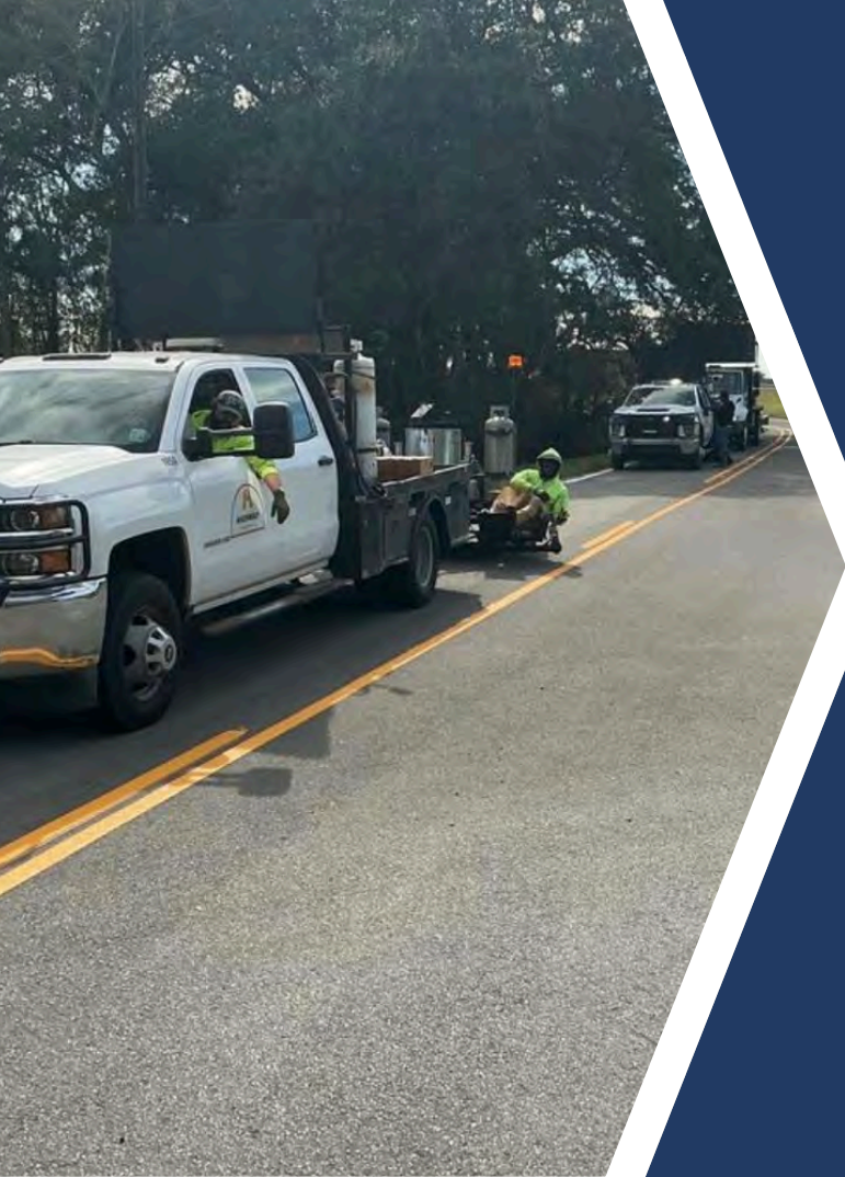
St. Mary Parish Signing and Striping Project - Pavement Striping Operations
