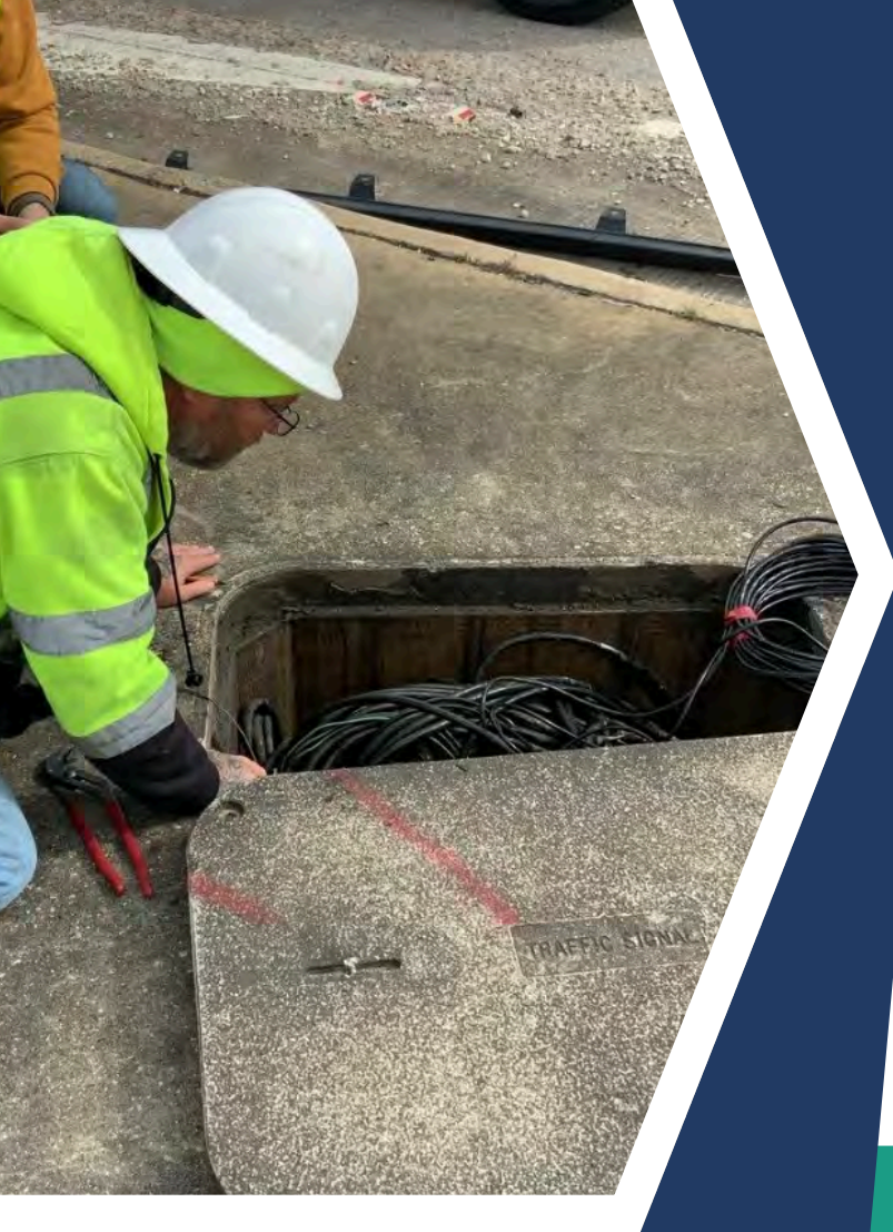
Lafayette FYA Project - Traffic Signal Inspection
