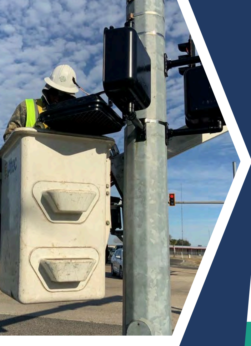
Lafayette FYA Project - Signal System Installation and Testing
