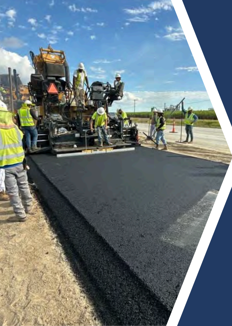
US 90 RR Overpass Project - Asphalt Paving Operations
