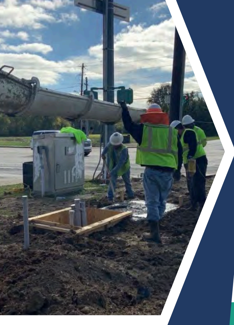
Signal Installation and Field Inspection - Lafayette, Louisiana
