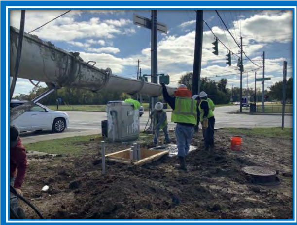
Signal Foundation Installation : Lafayette, LA
