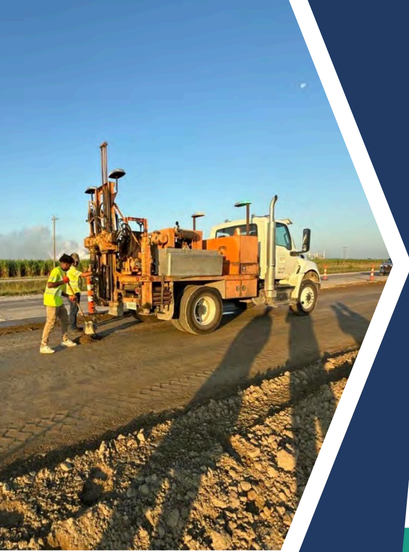
US 90 RR Overpass Project - Subsurface Drilling and Field Investigation
