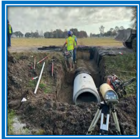
Drainage Installation & Utility Coordination
