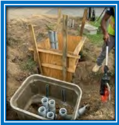
Signal Foundation Installation : Lafayette, LA
