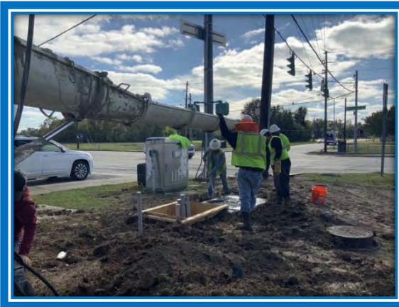
Signal Foundation Installation : Lafayette, LA
