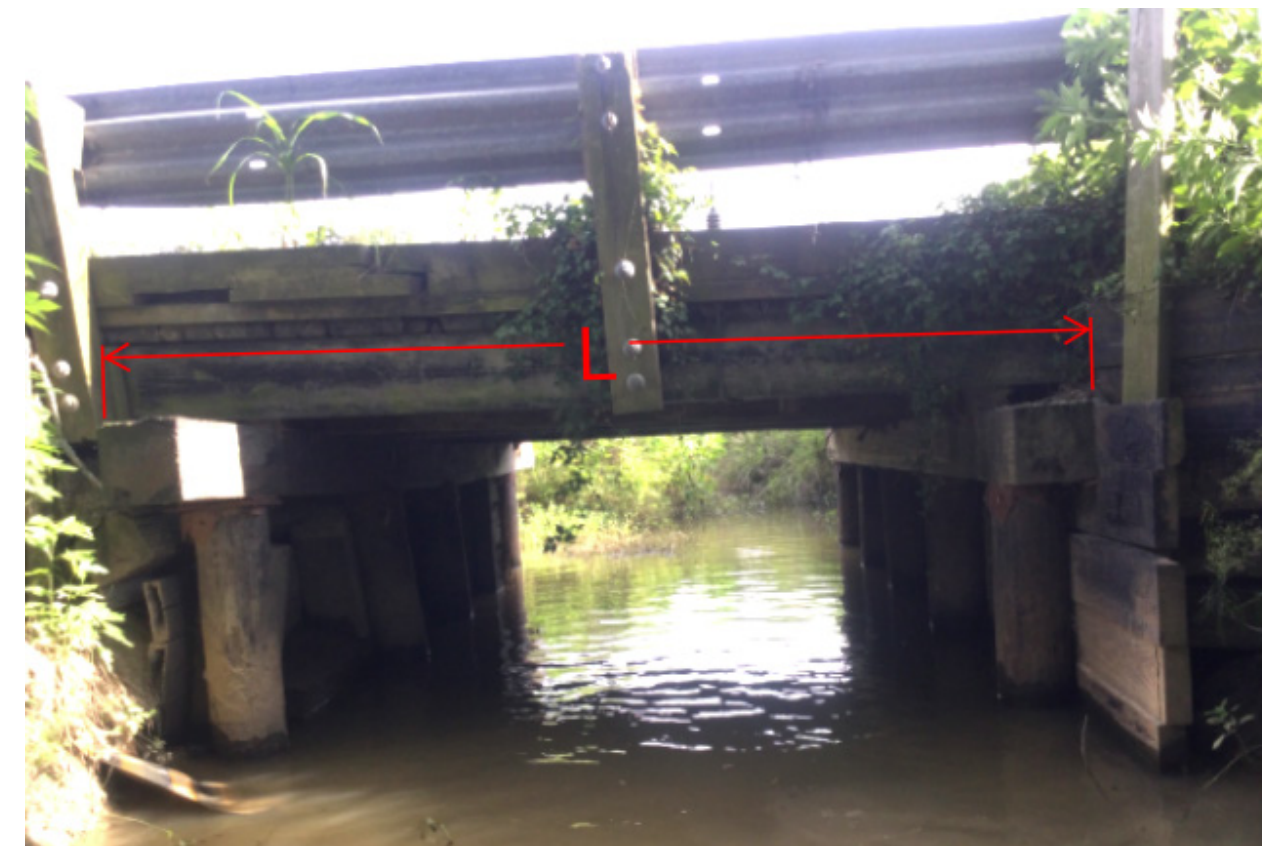
Single Span timber
