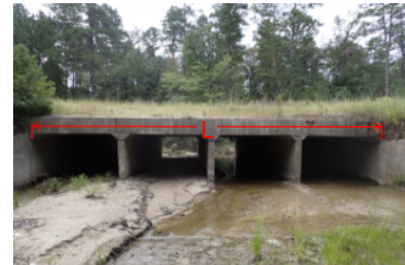
Multiple Span Curved Bridge 4-Barrel Reinforced Concrete Box Culvert
