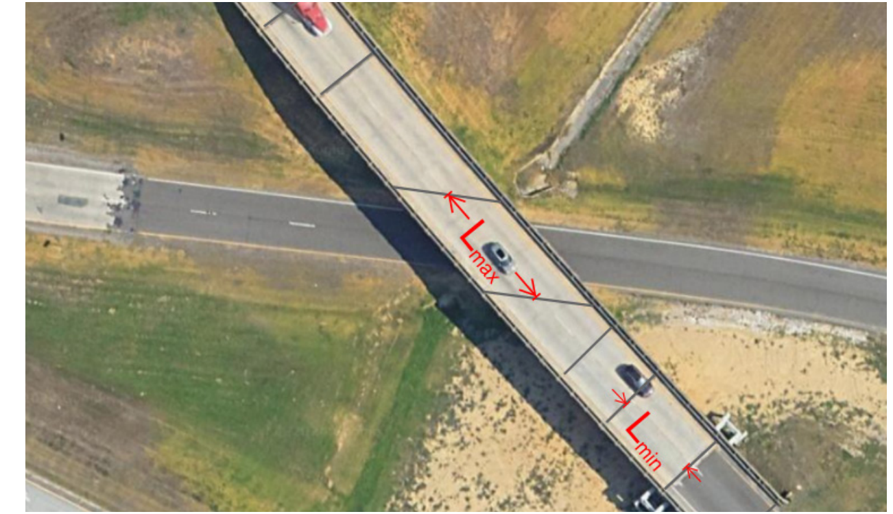
7-Span Steel Girder
