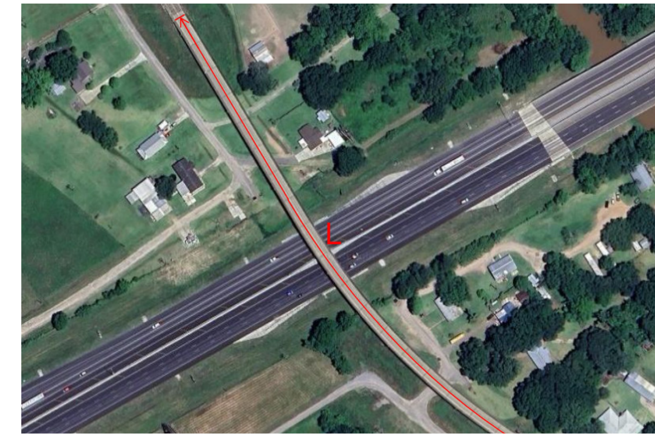
Multiple Span Curved Bridge
