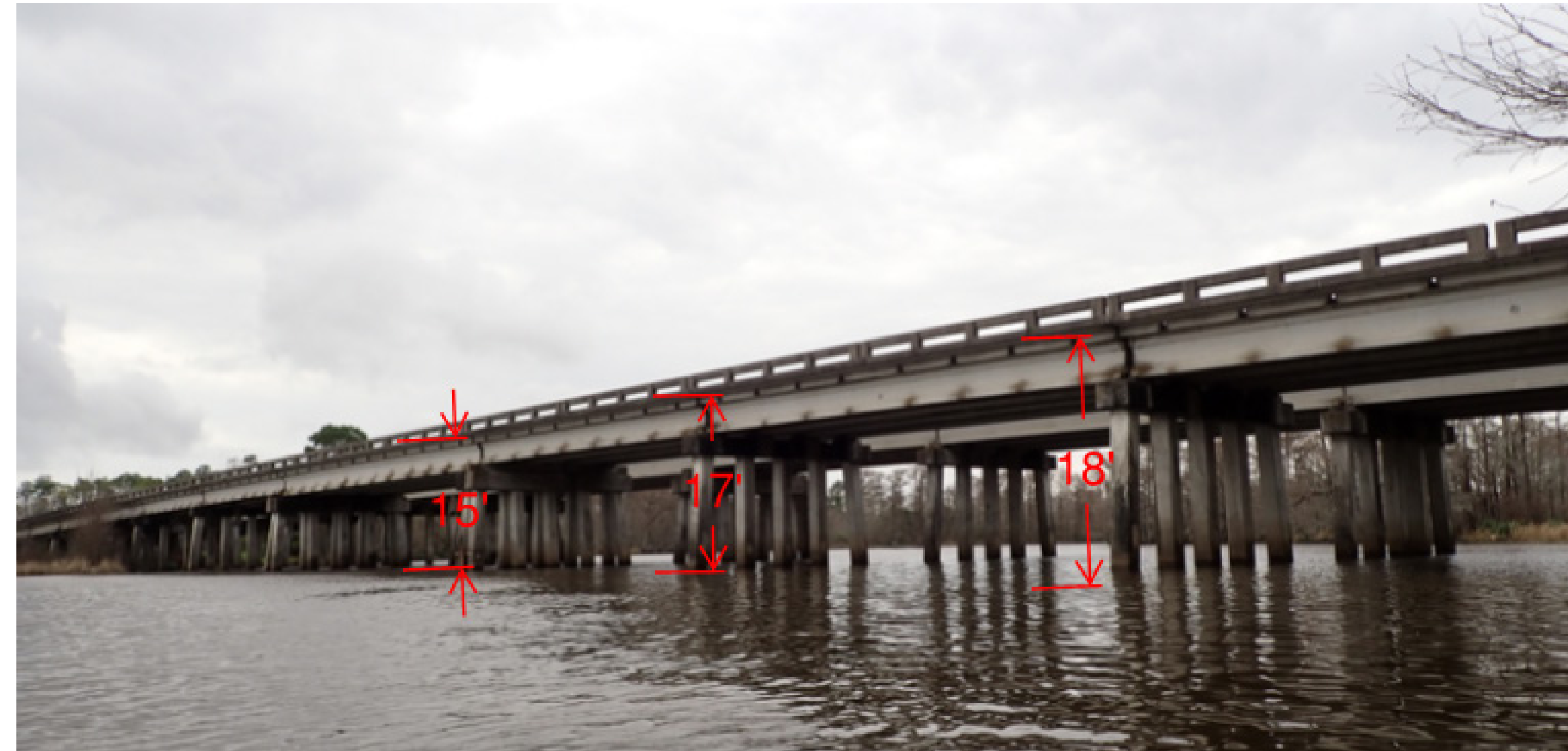
Maximum Bridge Height Example 1
