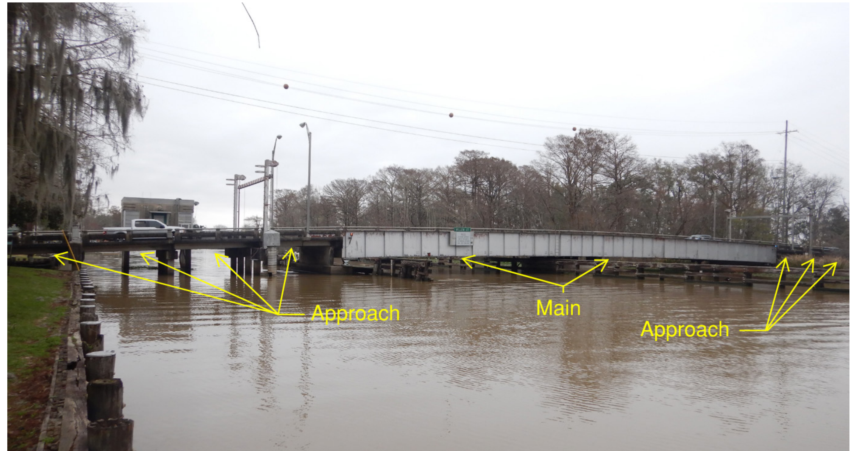
Photo 1: 2 Movable main spans and 7 slab span approach spans
