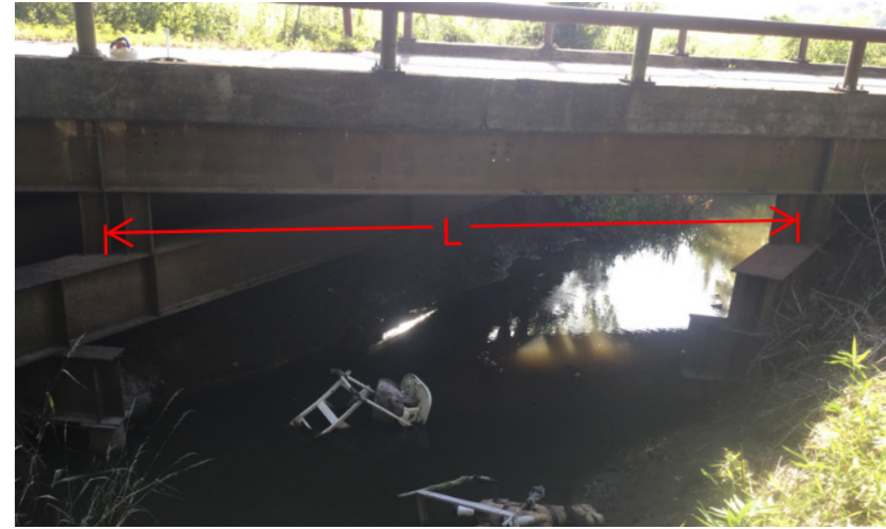
Single Span Steel Girder
