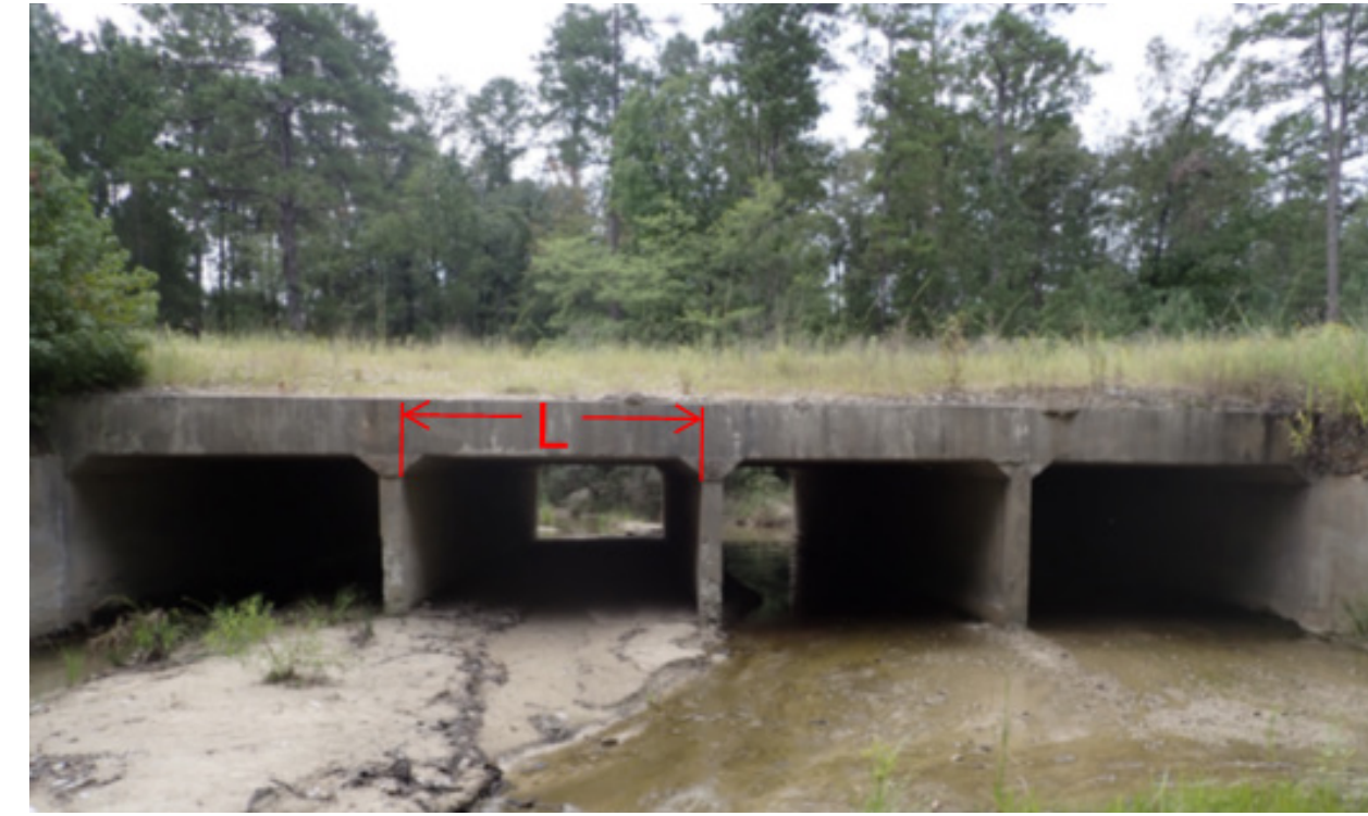
4-Barrel Reinforced Concrete Box Culvert
