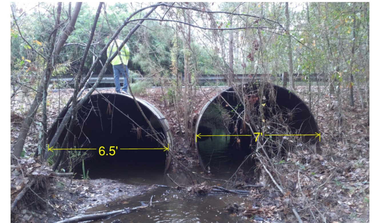
2-Span Corrugated Steel Culvert
