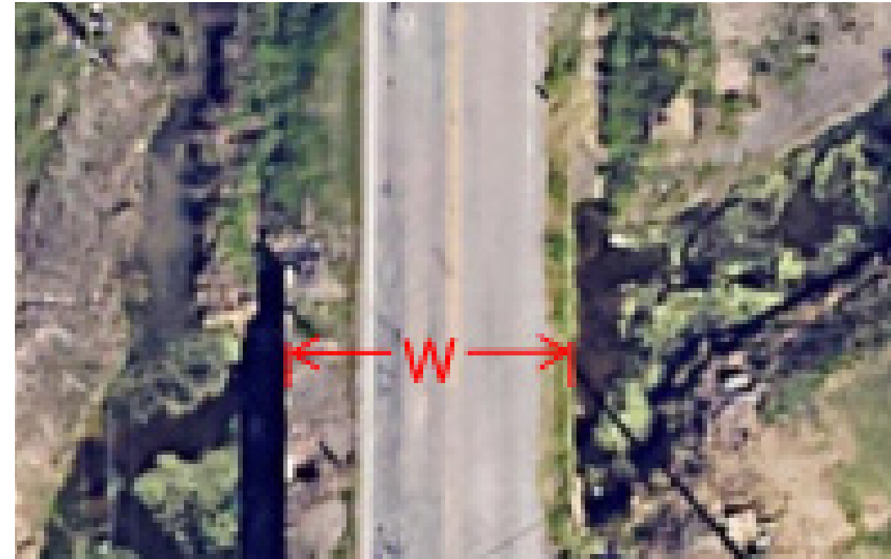
Reinforced Concrete Box Culvert
