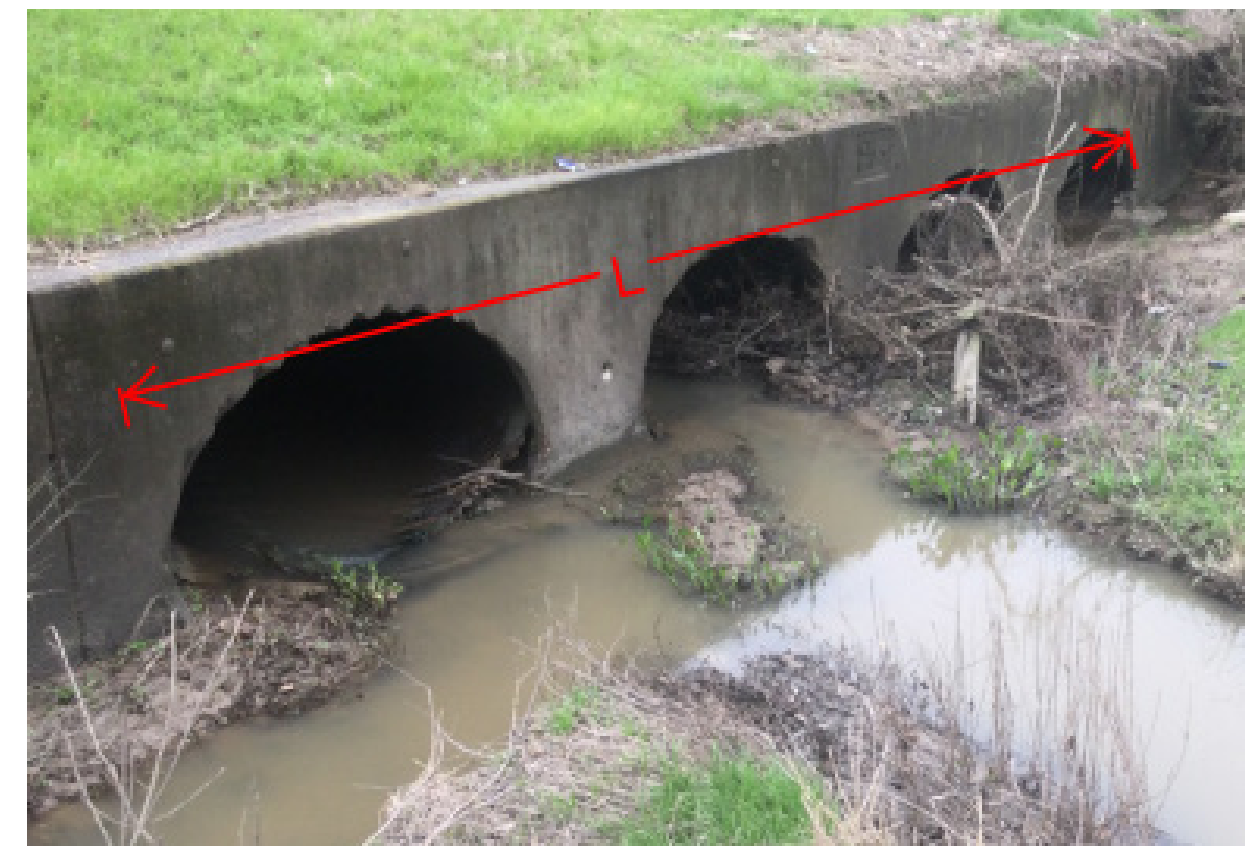
4-Barrel Corrugated Steel Culvert
