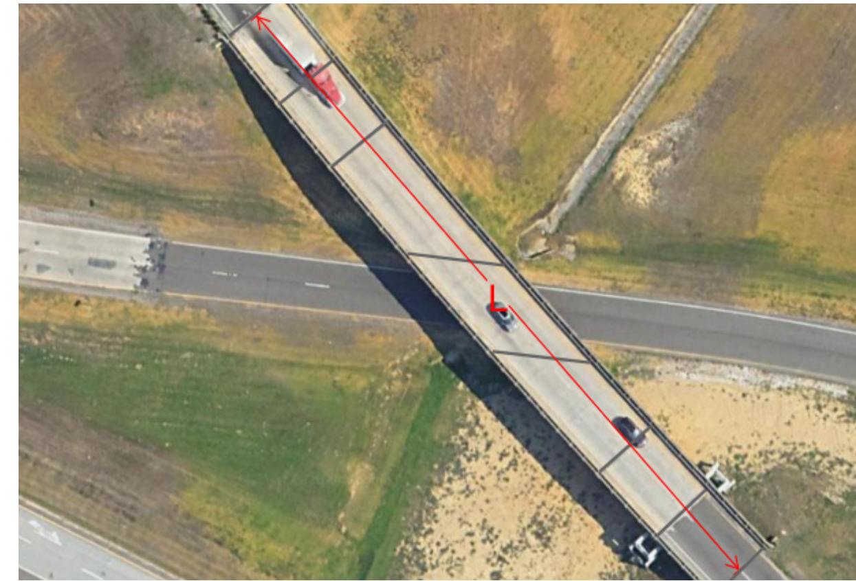
7-Span Steel Girder
