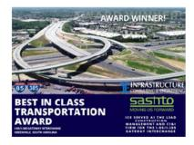
This Design-Build project involved interstate improvements consisting of reconfiguring a new interchange within the general footprint of the existing interchange by staging construction of the new lanes, ramps, and bridges while maintaining traffic. It also included widening of I-385 through the project limits and improvements were made to several local roads. Additionally,
