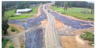
widened from two lanes to four lanes as it approaches the new roundabout. Providence personnel are providing Construction Engineering and Inspection (CE&I) services for Phase 4, Utility Relocation, and Phase 6, Construction, relative to the widening of LA 1026 (Phase I of the project); this includes construction project management, LA DOTD coordination, Site Manager-Materials, and 2059 Project Closeout.
