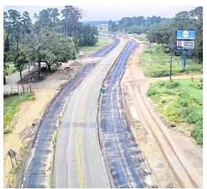
This project is under the LA DOTD CE&I IDIQ for District 62. The scope of this project aims to widen both US 190 and LA 1026 (Juban Rd.); installing drainage and curbing, milling, overlaying asphalt, and relocating all utilities within the corridor. Curb and gutter with subsurface drainage will be installed along Juban Road and US 190. The entire project will be constructed in two phases;
