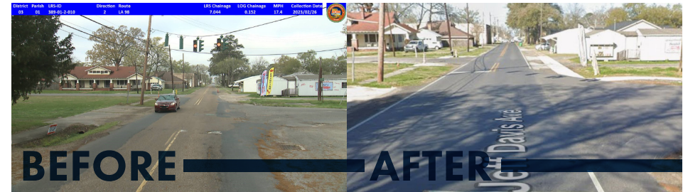
DISTRICT 03 LA 98 AT N POLK ST / CITY OF RAYNE LADOTD repaired LA 98. The improved roadway includes an improved intersection that had drainage and pedestrian issues.
