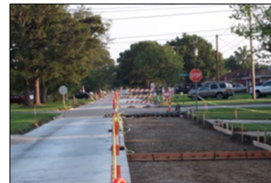
CONSTRUCTION IN PROGRESS HARVARD AVENUE
