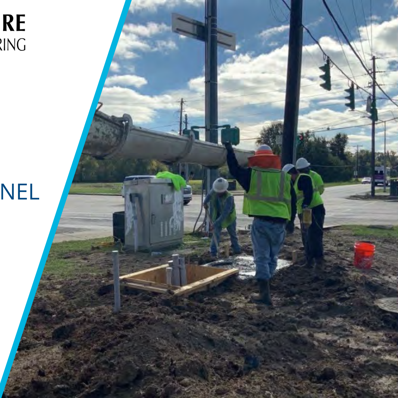
Signal Installation and Field Inspection
