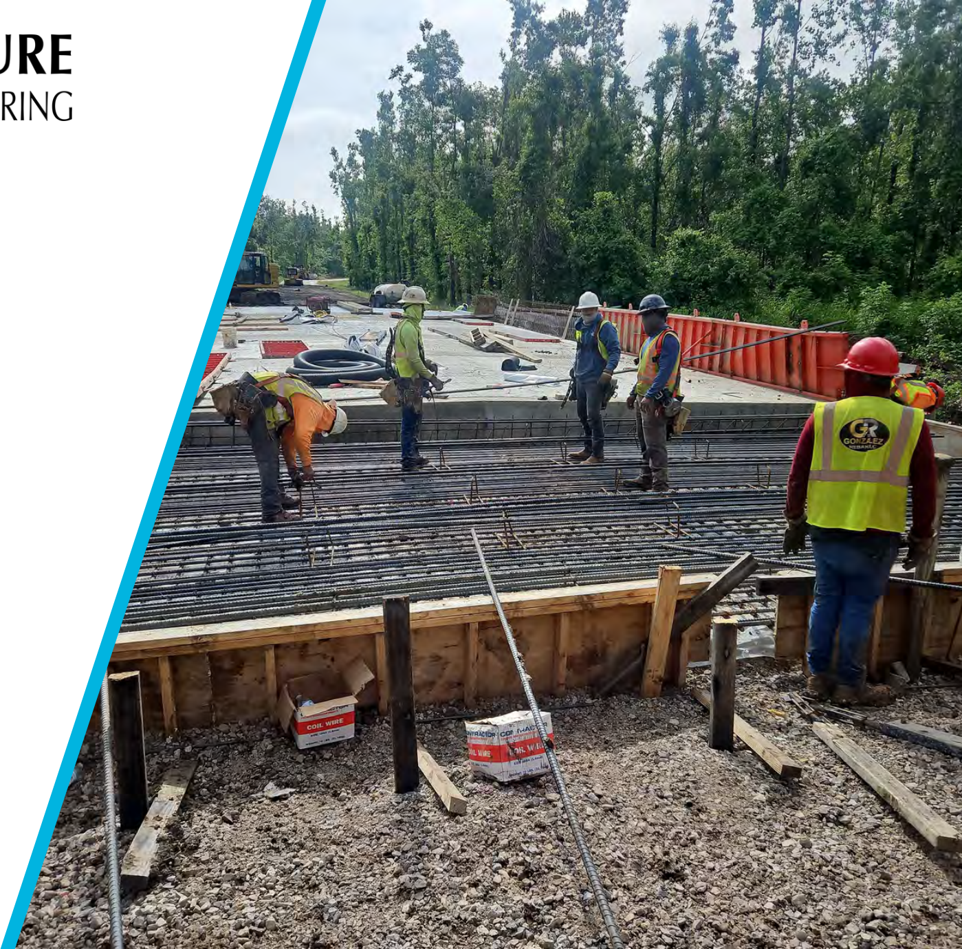
US 90 RR Overpass Project
