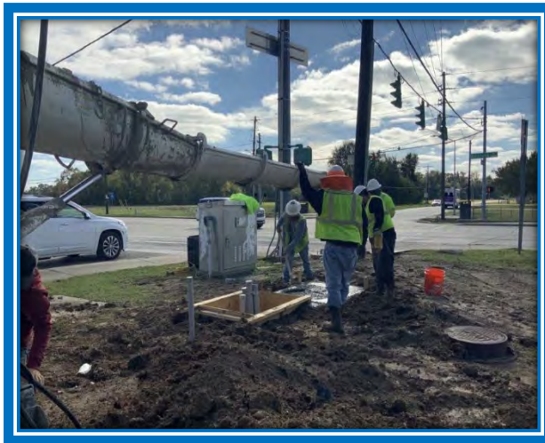
Signal Foundation Installation : Lafayette, LA
