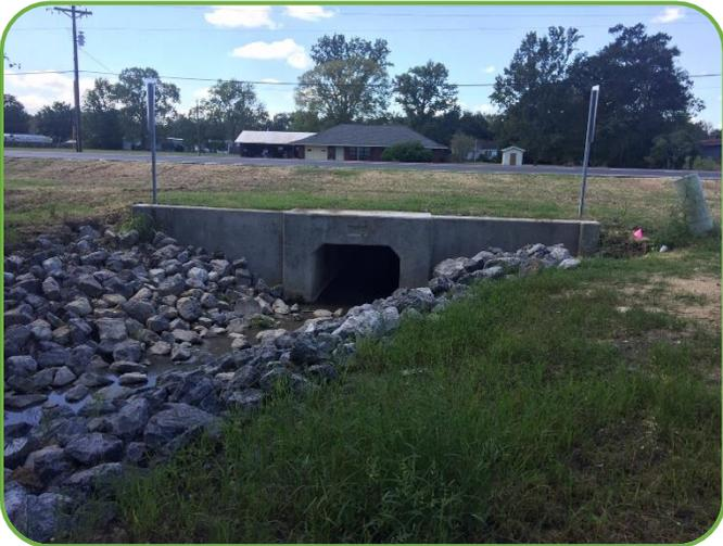
To accommodate the required amount of right-of-way per the DOTD design guidelines which would have severely impacted some businesses and would have caused their relocation. Meyer changed the design section in this area to subsurface drainage, which would fit within the existing right-of-way, thereby eliminating the need to relocate these business.
