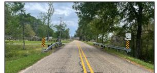
It is a two-span bridge with a precast concrete panel deck. barrier curbs and an asphalt overlay. It is supported on timber pile bents with timber caps, timber end bents and timber wingwalls:
