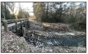
There is a set of three(3) gas pipelines passing diagonally under the Creek just north of the bridge, which is probably the reason for the streambed revetment:
