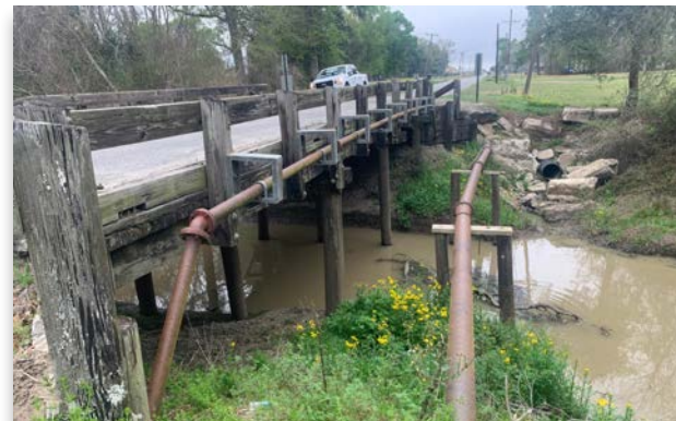
Photo showing water and sewer utilities along east side of bridge (site visit 3/11/22)
