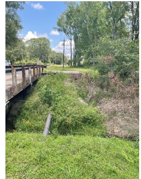
Photograph showing proximity of existing waterline to the south edge of the bridge.
