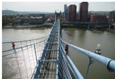
✚ NSTM and Element Level Inspection of John Roebling Suspension Bridge over Ohio River
