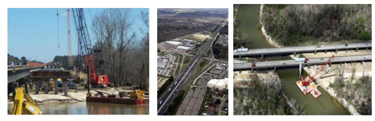
The project, from the O'Neal Lane/I-10 Interchange to Pete's Highway (eastbound) consisted of widening I-12 from 2-lanes in each direction to 3-lanes in each direction (6 lanes total) and reconstruction of the existing lanes. The additional lanes were constructed to the inside of the existing lanes (in the median) and a 12-foot width shoulder was constructed both inside and
