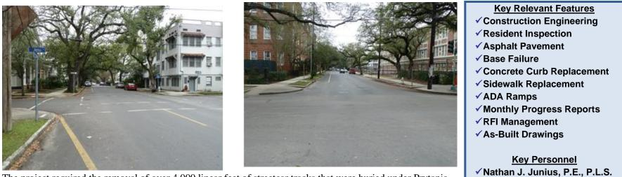
The project required the removal of over 4,000 linear feet of streetcar tracks that were buried under Prytania Street. The total project included over 4,000 linear feet of 35' wide **asphalt pavement, concrete curb replacement, sidewalk replacement and ADA ramps** which included a heavy duty concrete pavement with an underlying aggregate base course. The drainage system was replaced with 4,450 linear feet of 15" to 24"
