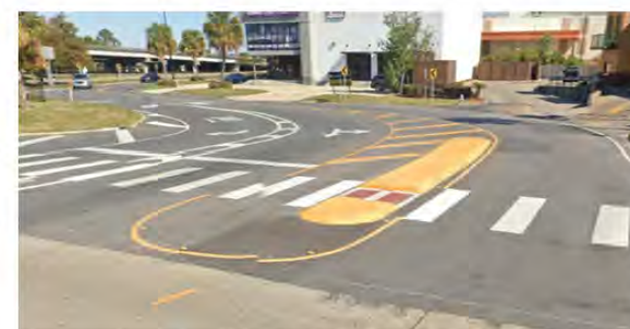
Figure: High visibility crosswalk and pedestrian refuge installed at I-10 Service Road and Read Boulevard
