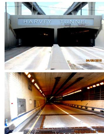
ECM's scope of services included, but was not limited to, field inspection with the project team; inspection of tunnel and approach pavements, tunnel walls, drainage, and portal buildings; report preparation support and reviews; and cost estimating.
