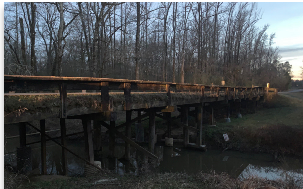
Photo showing profile of bridge and recent substructure repairs (site visit 3/1/22)
