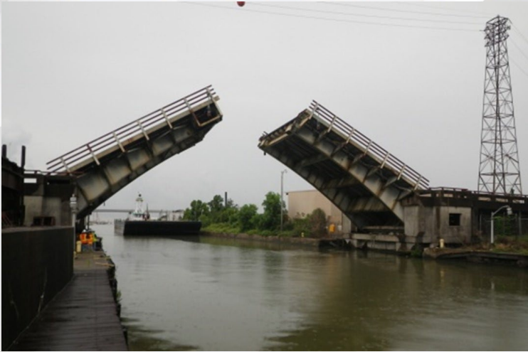
Figure 2: 4 th Street Bridge Opening (Modjeski and Masters, Inc.)
