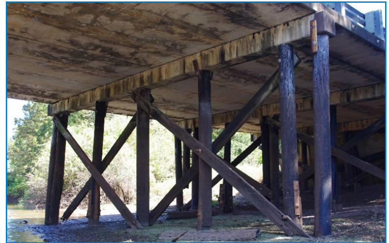
Deteriorated and Repaired Bent
