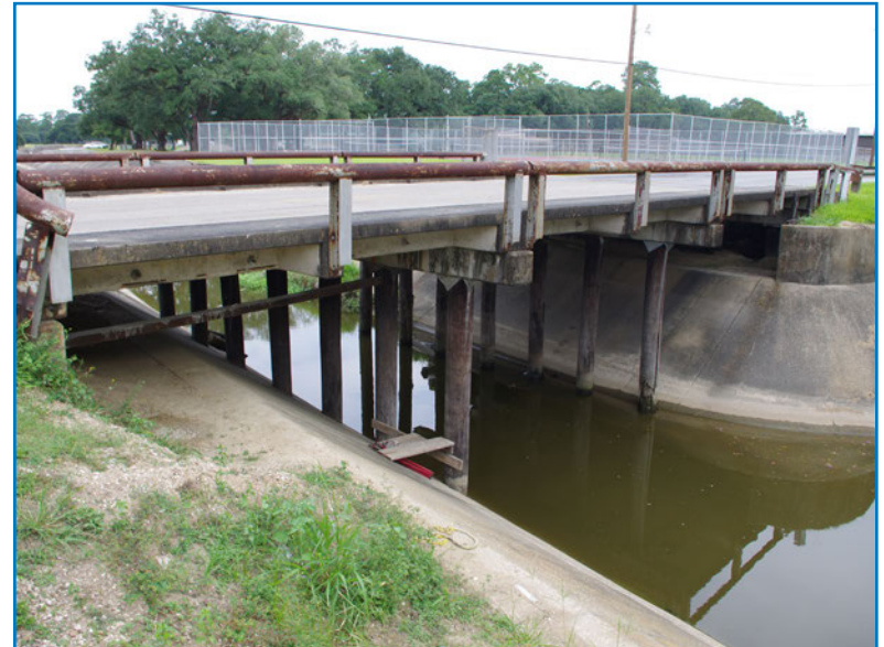
Example Slab Span Bridge Without Plans, 500 Bridges in total were load rated in the Task Order of similar type and complexity
