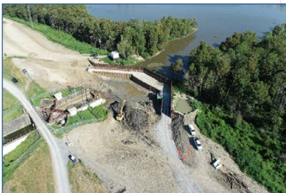
The construction contract was advertised as a bifurcated solicitation to accelerate procurement time.
