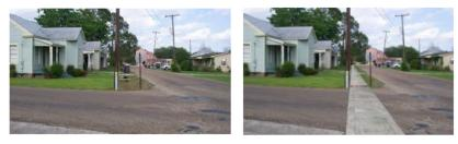
bricks at approximately twelve-foot (12') intervals helped to beautify the sidewalk. To be ADA-compliant, a truncated dome pattern was stamped into the concrete at the intersections. The City of Patterson took the initiative to install subsurface drainage in anticipation of the sidewalk being constructed. Providence personnel completed the DOTD-TAP application, headed grant administration activities, and provided QA/QC services. In addition, the team conducted
