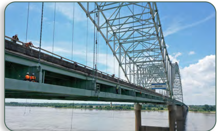
HNTB mobilized and performed emergency fracture critical member inspection and structural assessment in seven days for the Hernando de Soto Bridge for the ArDOT.
