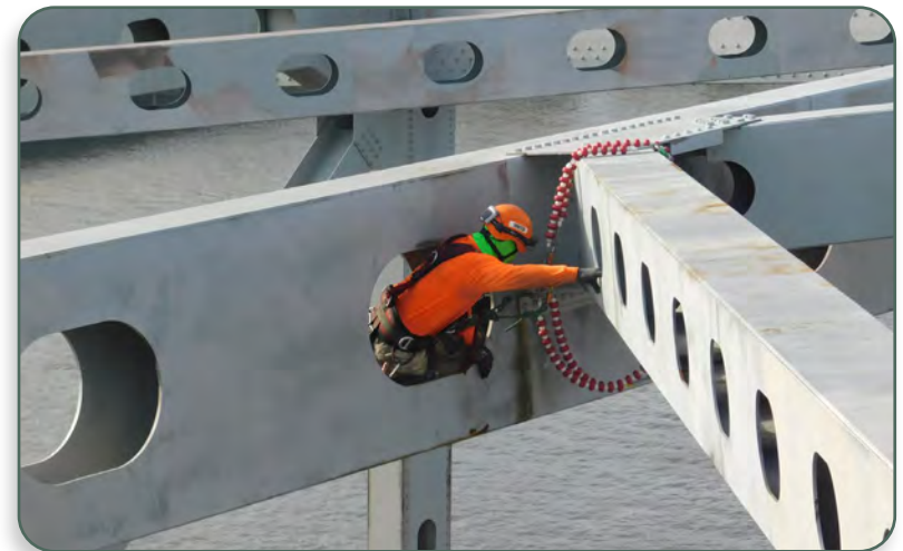
Rope access-trained inspectors were deployed with no lane closures to minimize traffic delays, reduce costs and meet schedule.
