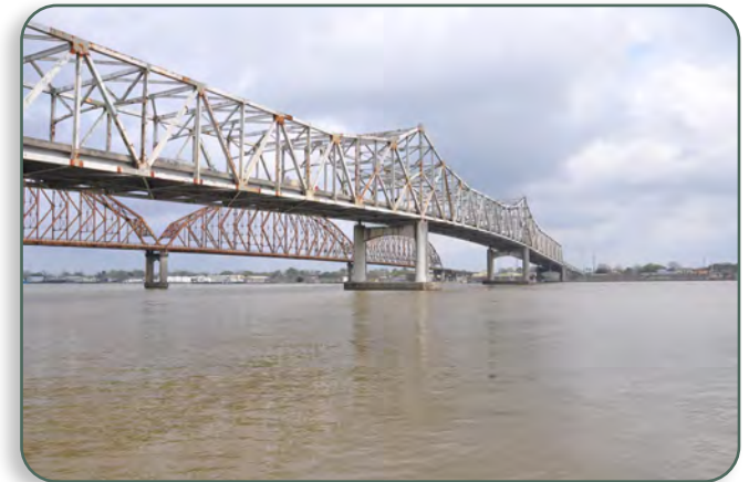
Inspection included ultrasonic testing of fracture critical pins, and coating corrosion assessment
