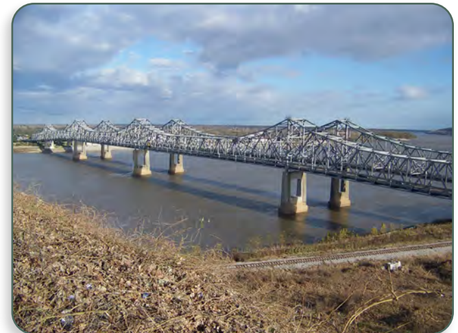
HNTB developed a procedure to temporarily restrain the joints, bypass the load off the pin and link, remove the existing pins and link, line bore through the existing gussets, and install new a new link and pins
