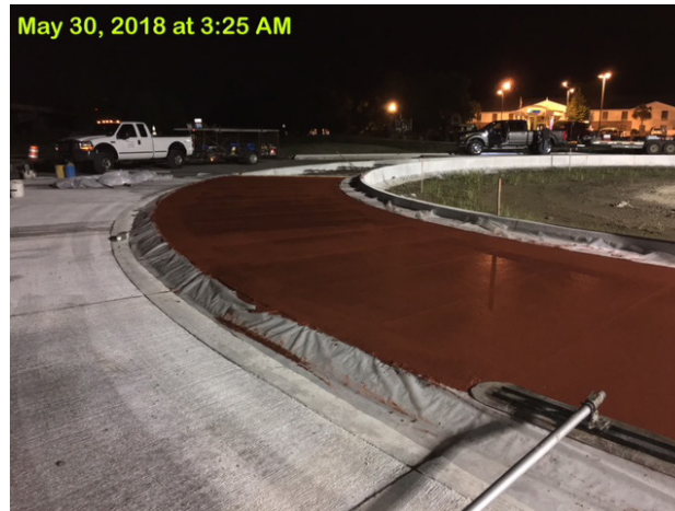
CE&I of colored concrete roundabout construction at the intersection of I-10 and LA 347
