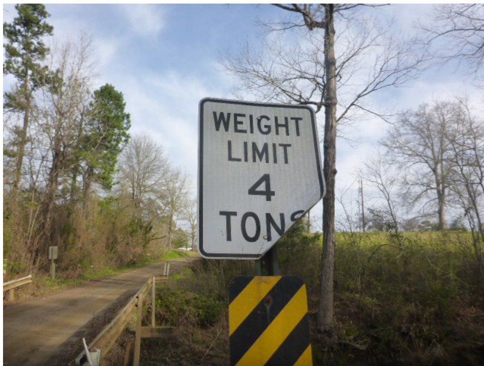
Figure 3-11: Damaged and incorrect weight limit sign
