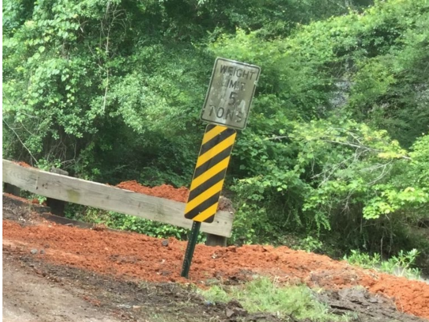
Figure 3-12: Illegible weight limit sign
