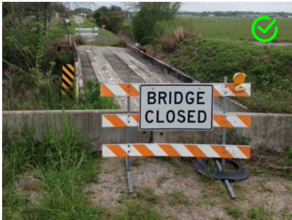
Figure 3-3: Correct closure with Type 3 barricade and concrete barrier
