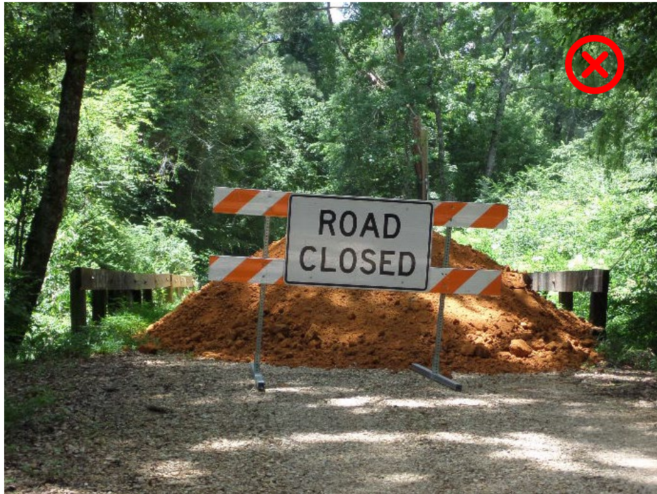
Figure 3-7: Incorrect closure using dirt pile
