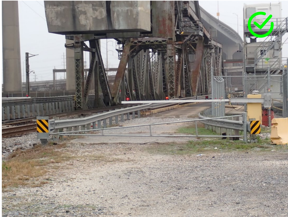
Figure 3-4: Correct closure with a locked gate
