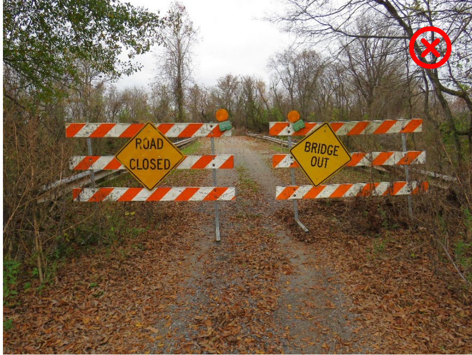
Figure 3-6: Incorrect closure with only Type 3 barricade. NOTE: Signage should not be mixed
