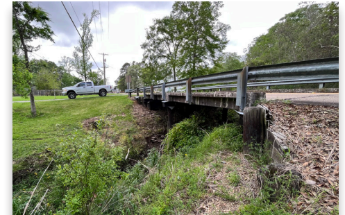
Looking west showing bridge, utilities and creek skew Site Visit - (4/2/2025)
