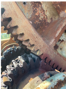
H&H performed NBIS inspections of Calcasieu River Bridge at West Fork
