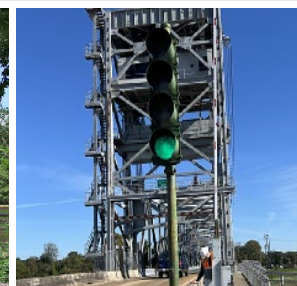
Jackson St Lift Bridge
