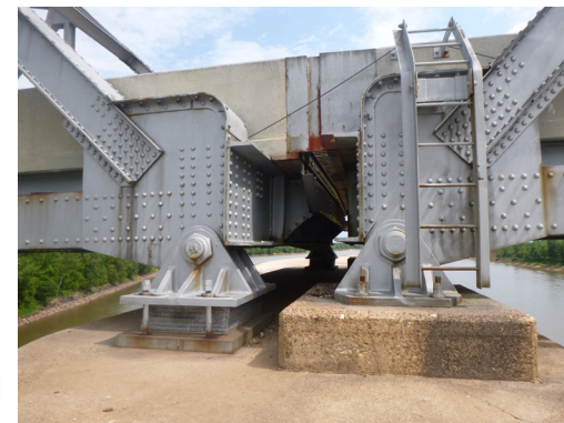
H&H performed NBIS inspections of Red River Bridge at Miller's Bluff
