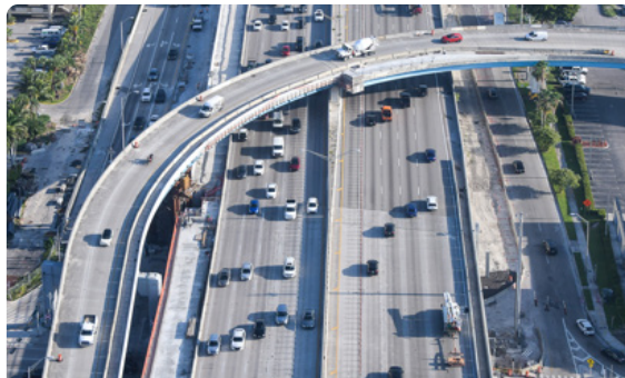
H&H provided the expedited design for the widening & resurfacing of the SR 826 Palmetto Expy and frontage road improvements.
