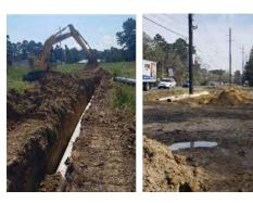
This project is under the LA DOTD CE&I IDIQ for District 62. The scope of this project aims to widen both US 190 and LA 1026 (Juban Rd.); installing drainage and curbing, milling, overlaying asphalt, and relocating all utilities within the corridor. Curb and gutter with subsurface drainage will be installed along Juban Road and US 190. The entire project will be constructed in two phases;
