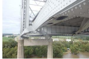
with the project surveyor, WJE engineers used their laser scanning data to assist in restoring the structure's geometry. Other project responsibilities assumed by WJE included development of jacking frame shop drawings, review of the replacement chord design, technical assistance during jack system installation, oversight of chord jacking operations, and instrumentation and monitoring of the truss.
