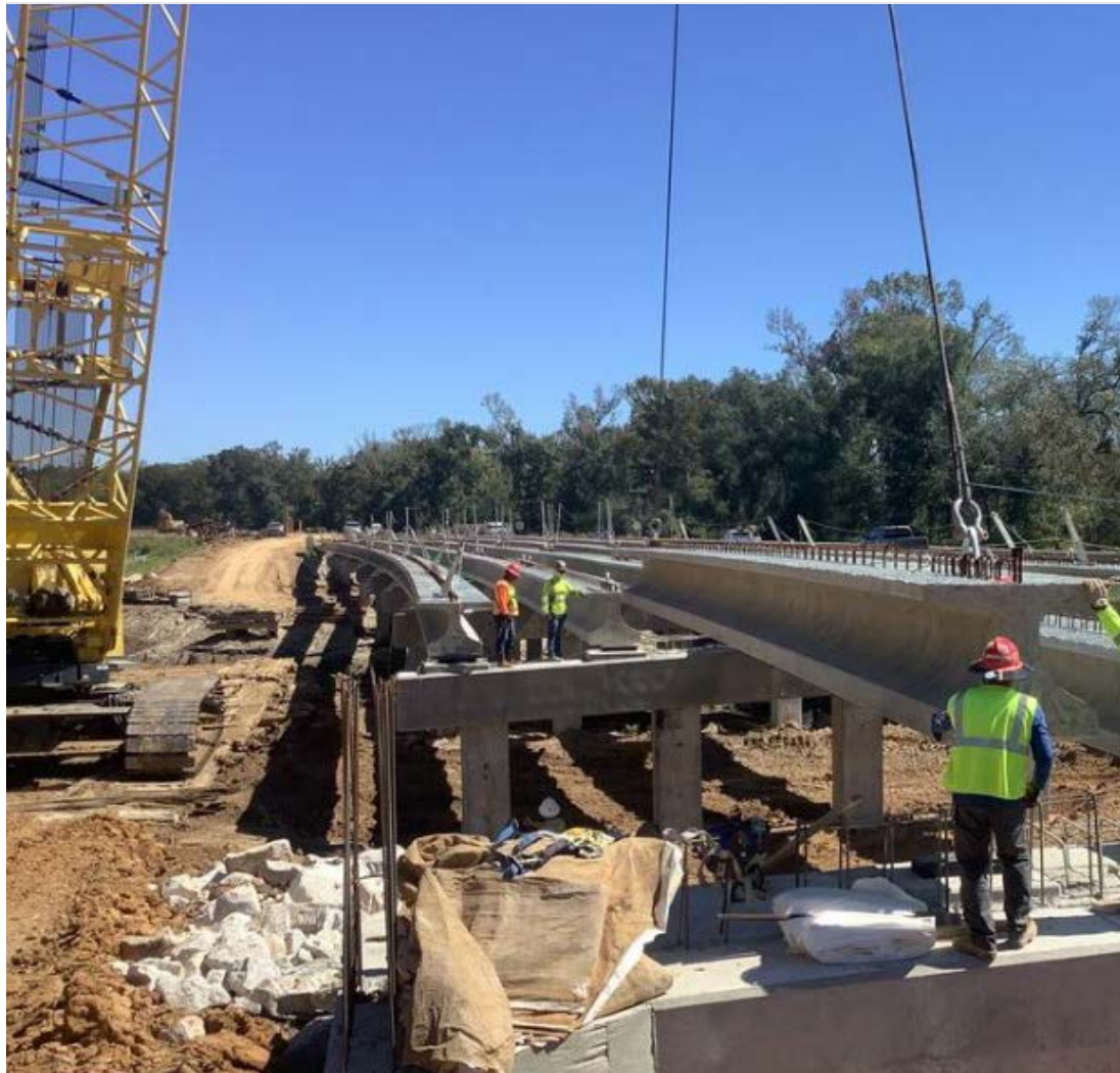
Bridge replacement being constructed by DOTD
