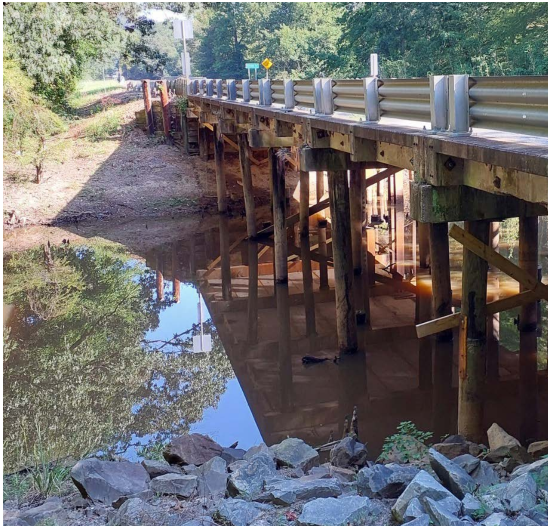
Current state of bridges near Shongaloo
