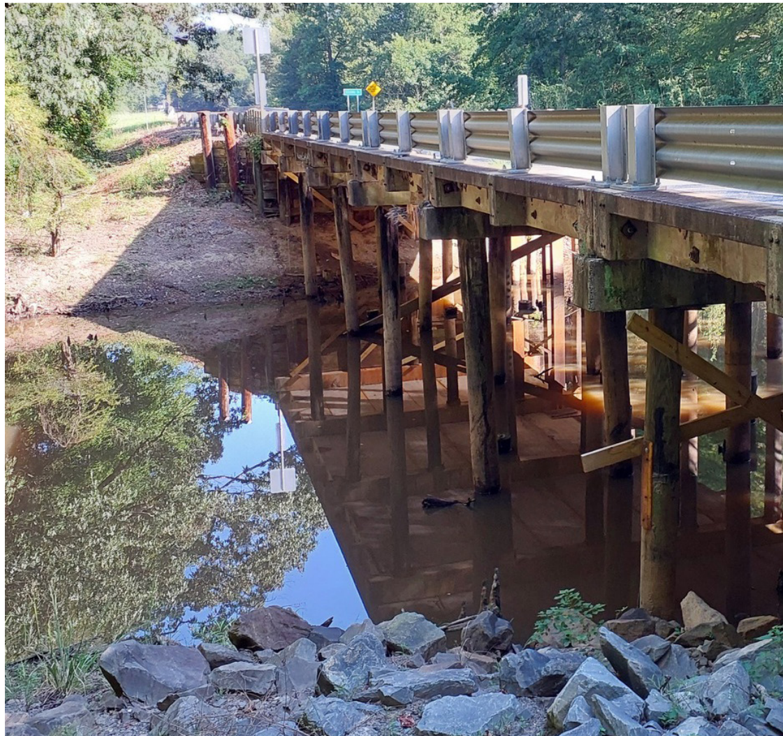
Current state of bridges near Shongaloo
