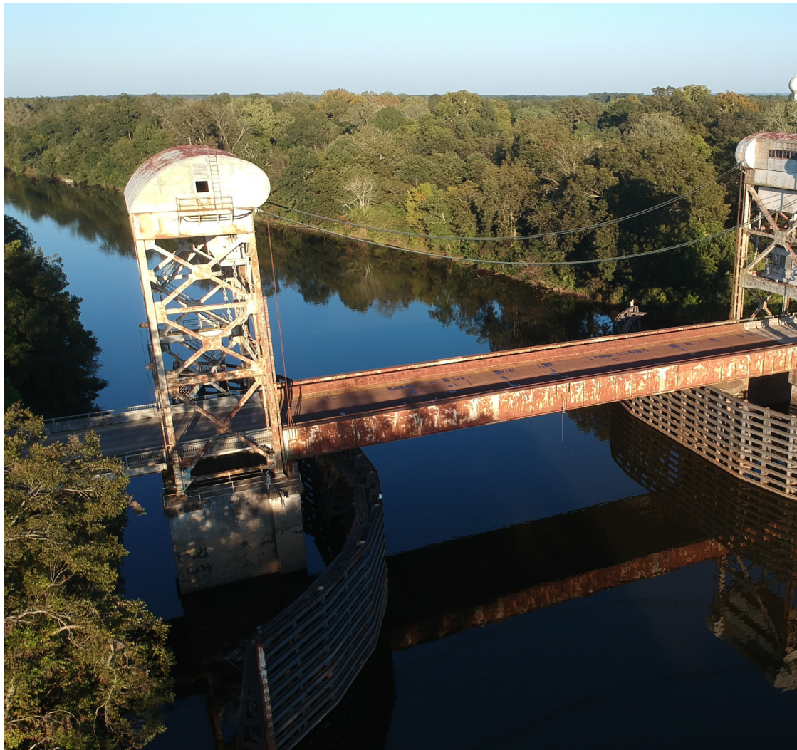
Tensas River Bridge at Clayton (Photo Credit: Louisiana Trust for Historic Preservation)
