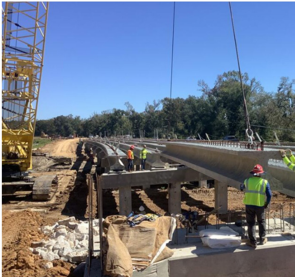
Bridge replacement being constructed by DOTD
