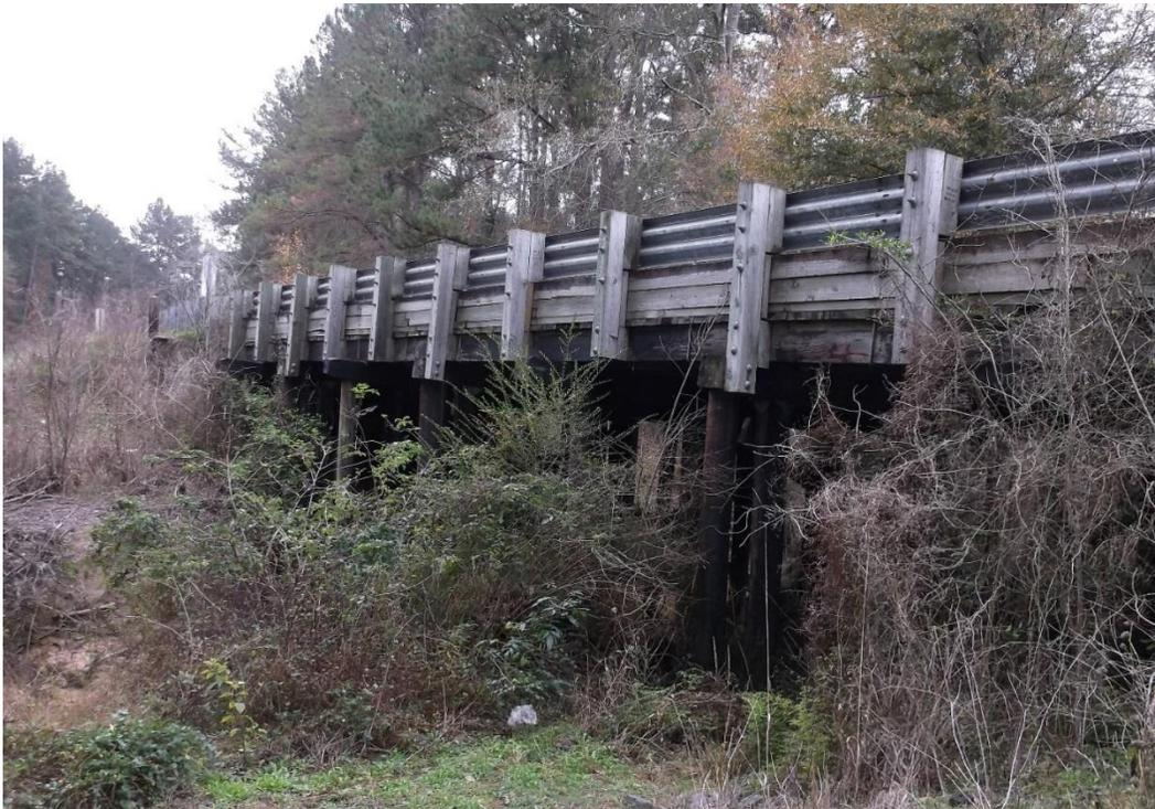
*Figure 10. Bridge 041090 in Rapides Parish, 1940. Example five or more spans – 16 spans comprising 78 feet.*
