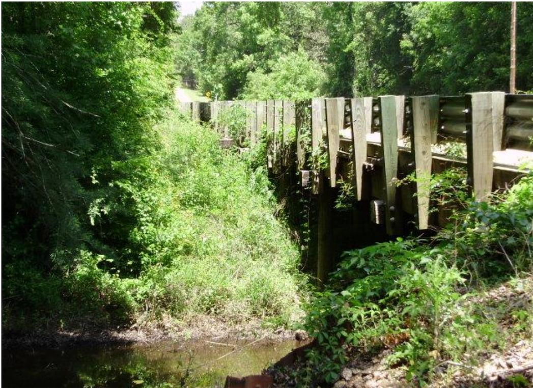
*Figure 4. Bridge 037640 in Grant Parish, 1931. This is the longest example in the study pool – 24 spans comprising 457 feet. See Figure 5 for another view.*
