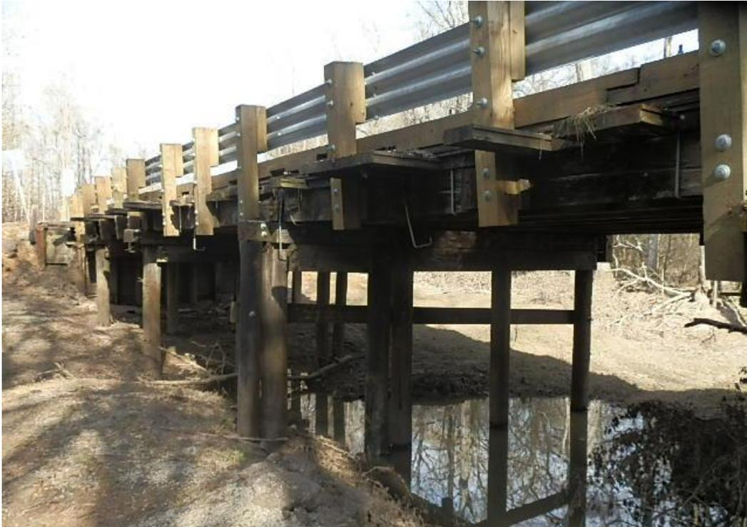
*Figure 11. Bridge 047070 in Caldwell Parish, 1931. Example with five or more spans – five spans totaling 97 feet.*
