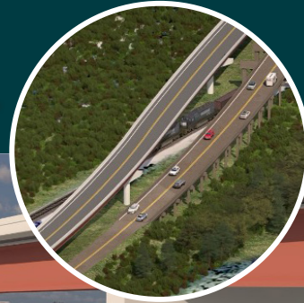
PHASE 1 NEW SOUTHBOUND BRIDGE CONSTRUCTION PARALLEL TO EXISTING BRIDGE
