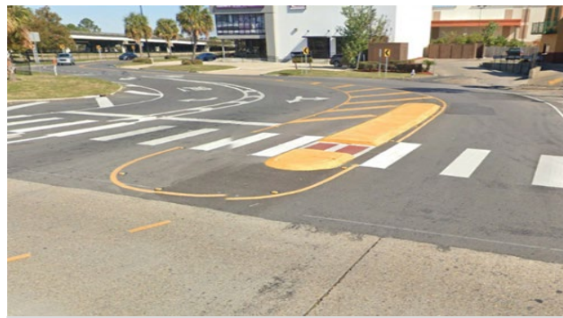
NO Ped Study: Implemented low-cost safety improvement on Read Blvd High-Visibility Crosswalk and Refuge Island
