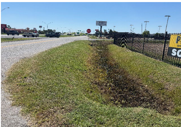
Figure 1 - Ditch Proximity to Service Road north of Reese Street
