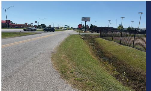
Ditch Proximity to Service Road North of Reese Street
