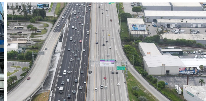
SR 826 over Metrorail
