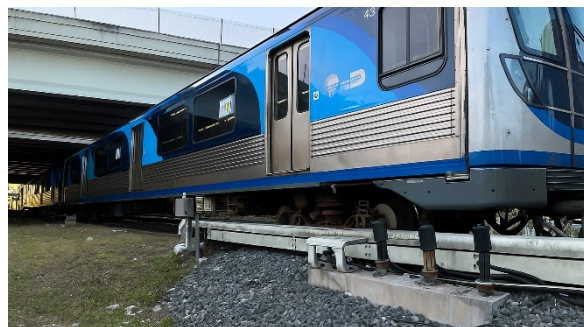
Metrorail under SR 826
