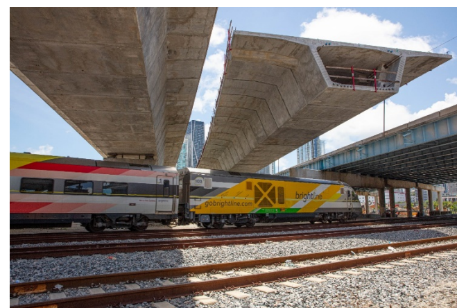
Brightline Rail Crossing under I-395
