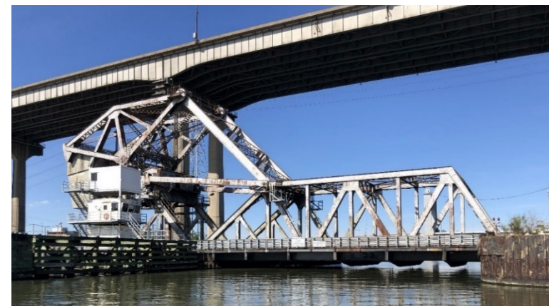
Almonaster Ave Bridge over the Industrial Canal
