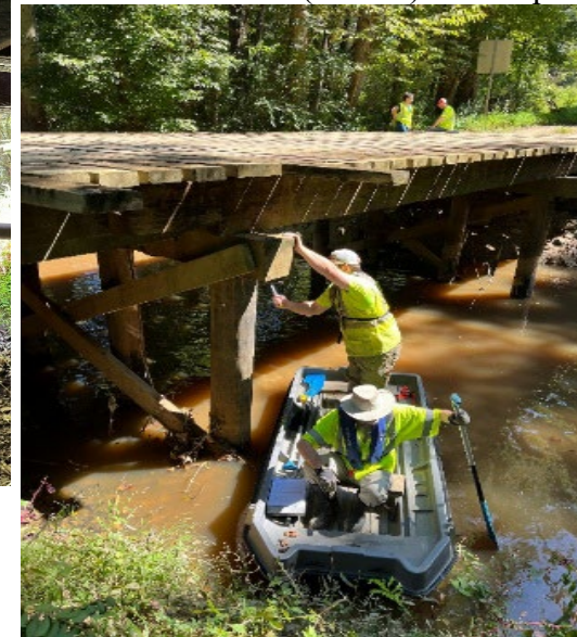
Tension Member (NSTM) and repair
